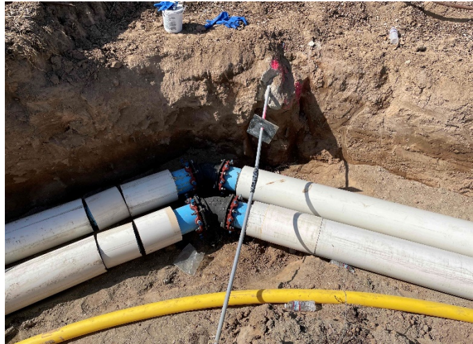
Installation of New Chilled Water Lines
