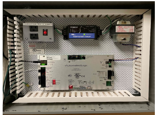
New HVAC Controls Installed
