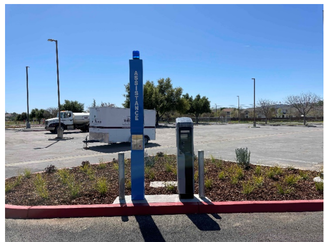
New Emergency Blue Phone and Permit Pay Station in Parking Lot 10.
