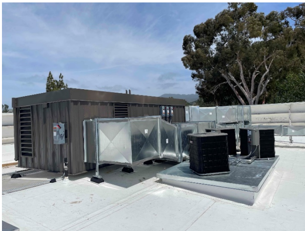
HVAC Equipment and Ductwork Completion on the 4100 Building
