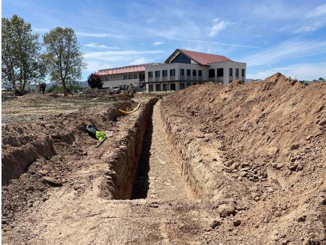
Trenching for Underground Site Utilities
