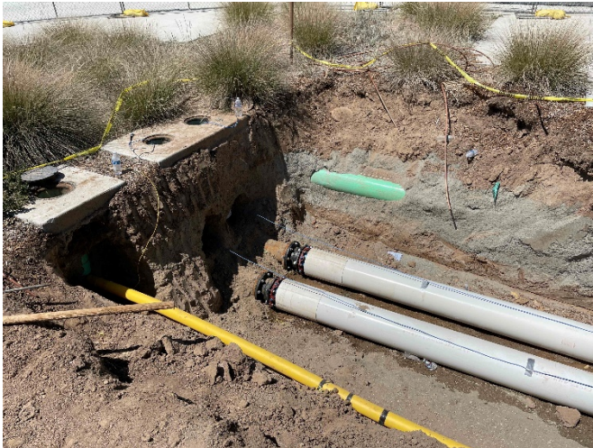
Installation of New Chilled Water Lines
