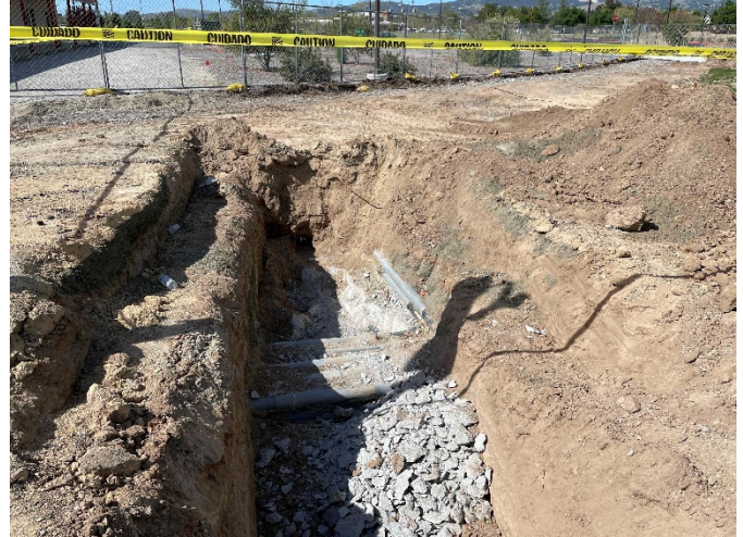
Trenching and Exposing of Existing Underground Utilities to be Extended
