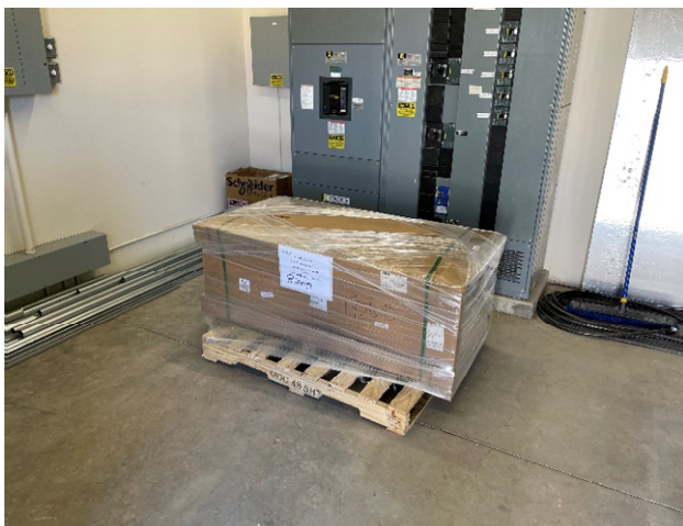
Delivery of the ATS awaiting installation
