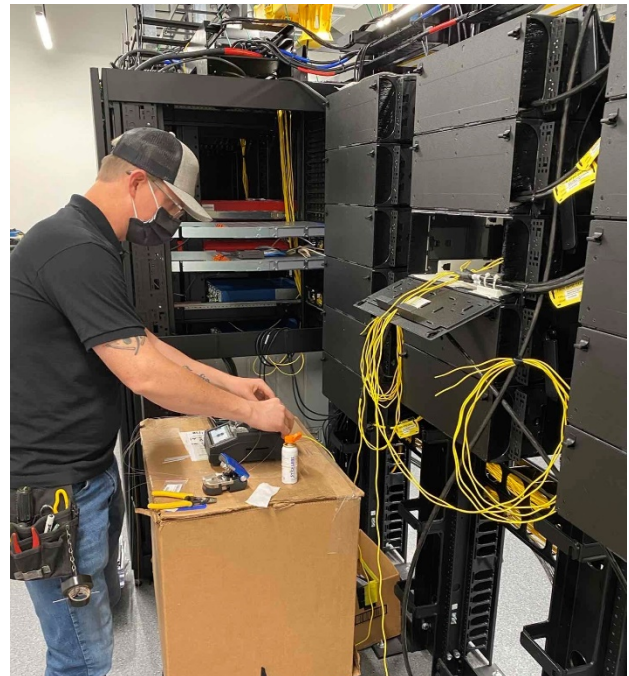
Installation of new Cat 6a cabling
