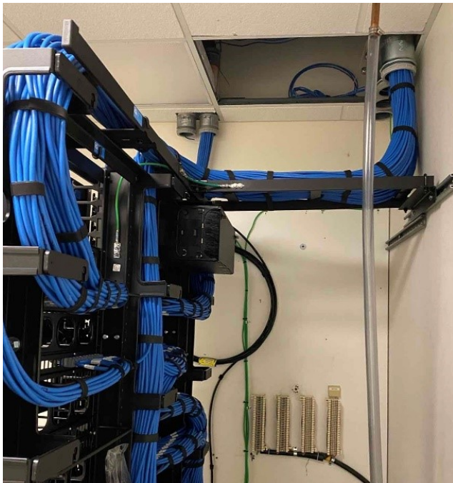
Installation of new Cat 6a cabling
