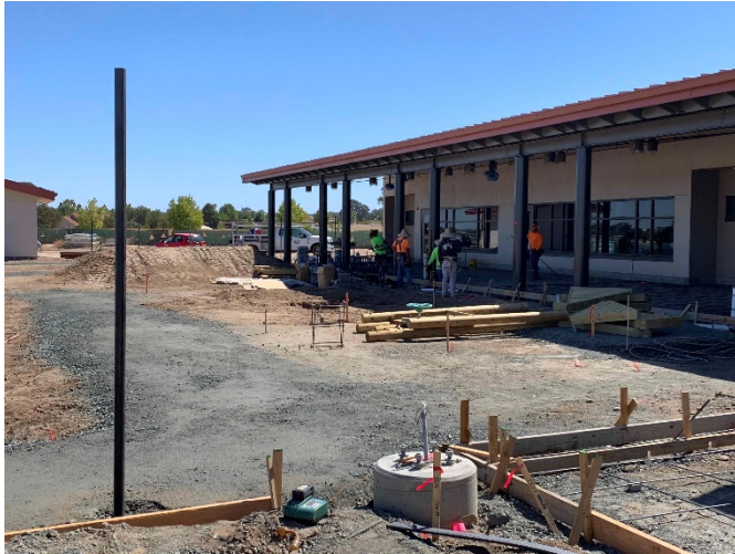
Play Area Sitework Progress
