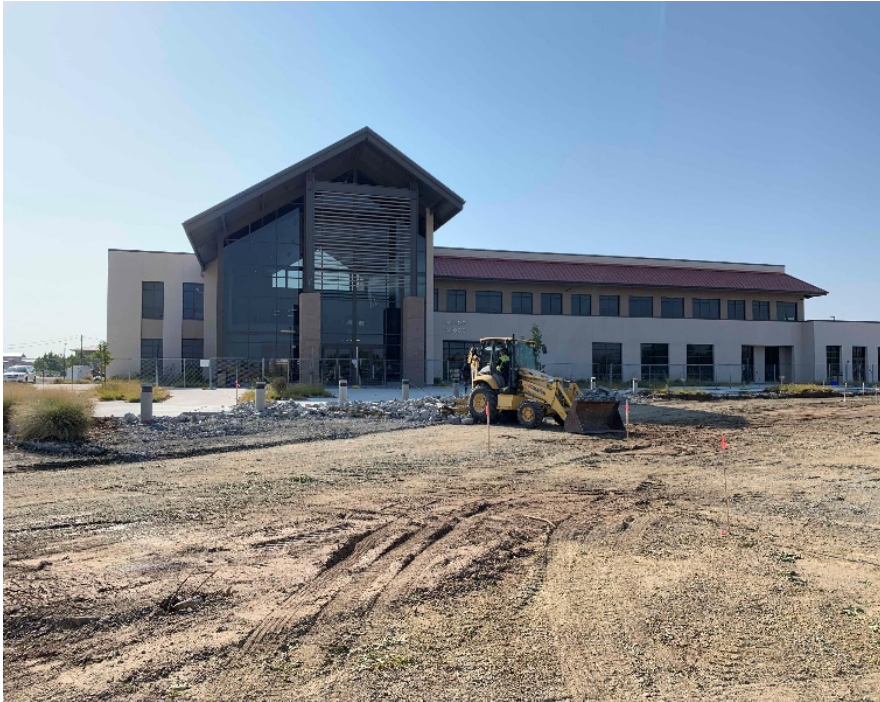
Sitework Demo Progress at Campus Center main entry
