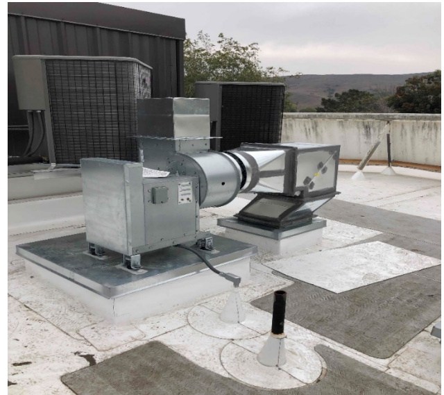
Finished installation of the Exhaust Fans on the 2200 Building
