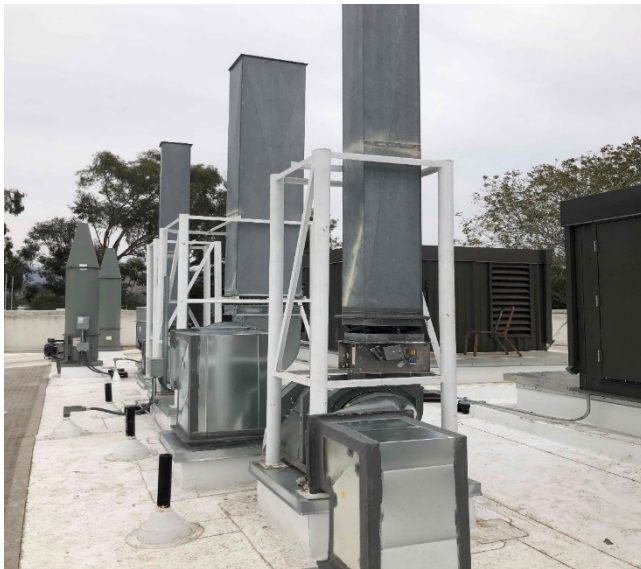
Finished installation of the Exhaust Fans on the 2200 Building
