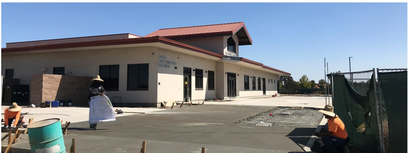
Site Concrete Progress at the Main Entrance
