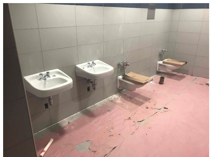
Bathroom Tile and Plumbing Fixture Installation Progress
