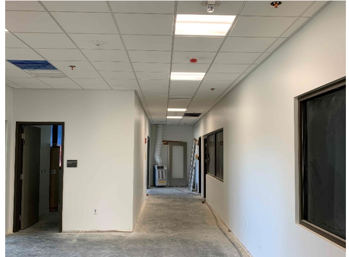
Acoustical Ceiling Tile Progress
