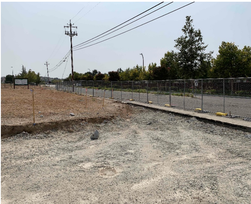
Sitework Progress at new Campus Entry drive approach
