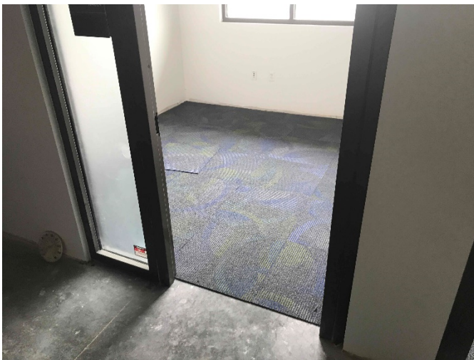
Carpet Installation at Offices
