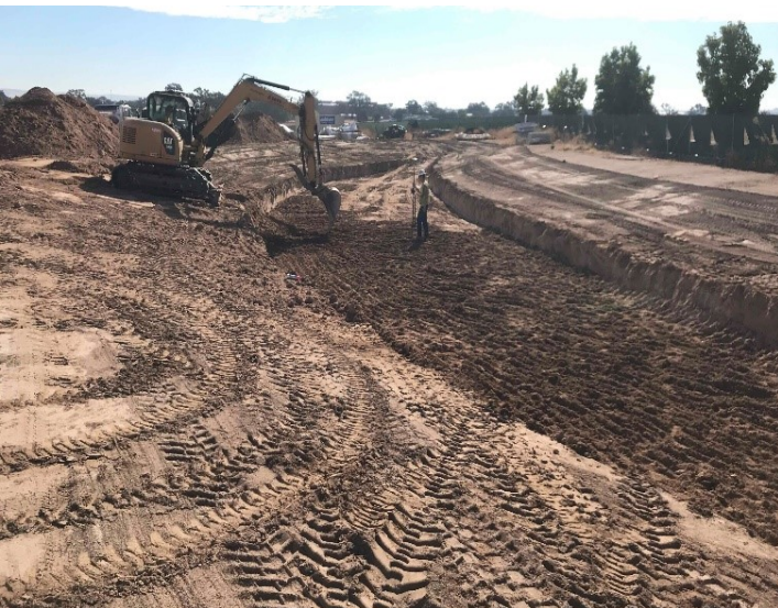
Site Grading Progress
