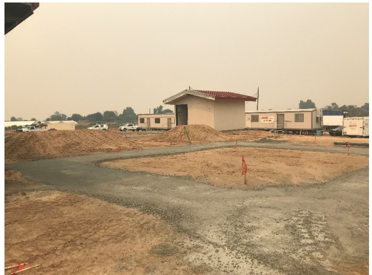
Exterior Play yard Sitework Progress
