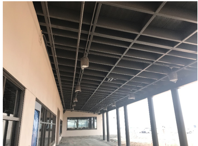
Covered Play Area Progress
