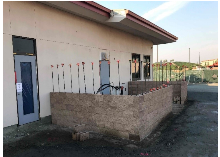
Transformer Yard Progress
