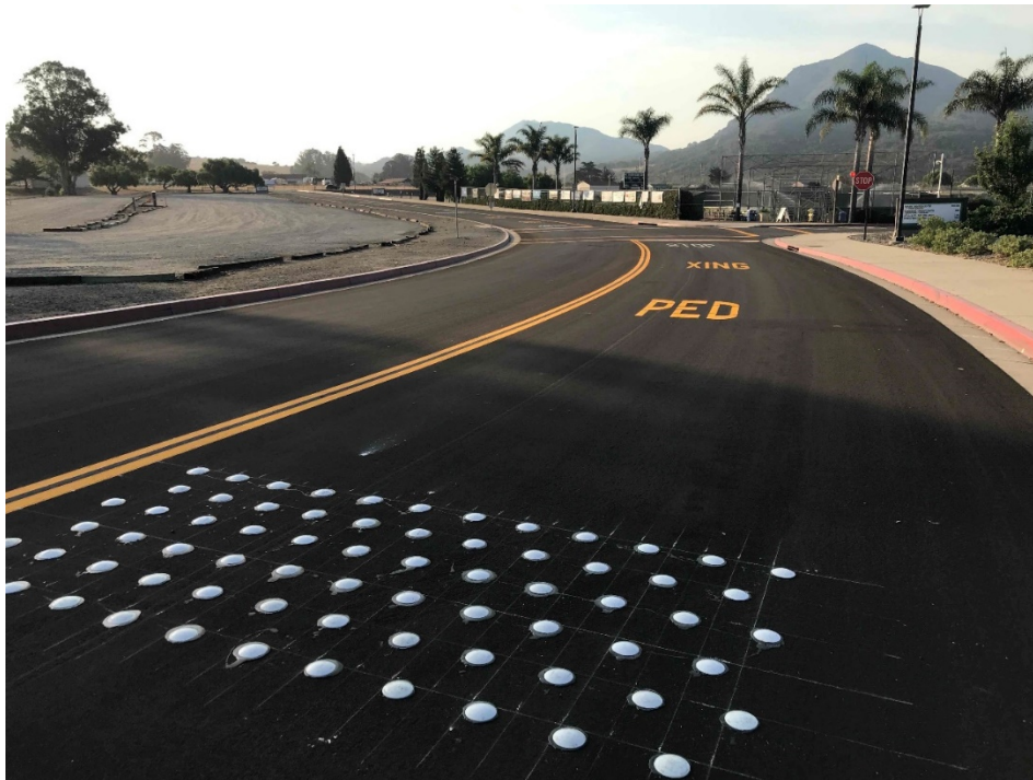
Completed Slurry Seal, Bump Stops and Striping on Romauldo Road
