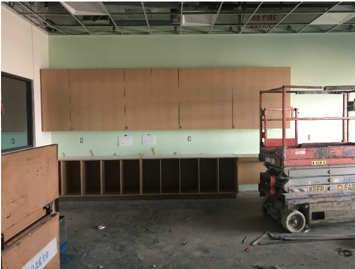
Casework Installation Progress
