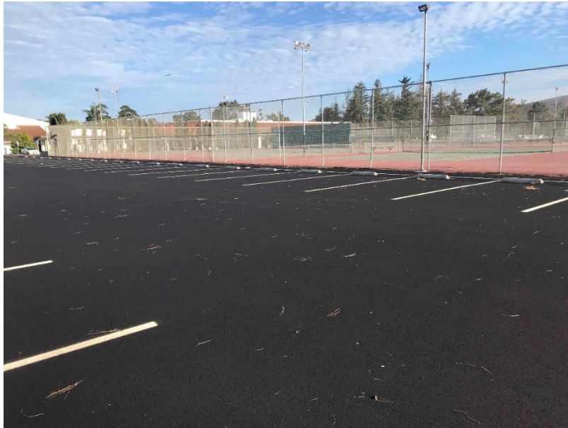
Asphalt and Striping Complete at Lot 6
