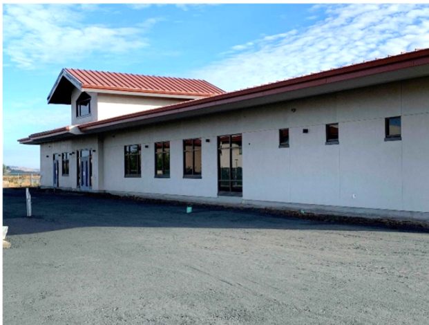
Plaster and Finish Paint Complete
