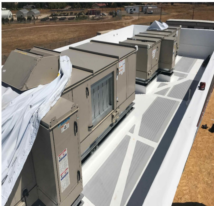
Membrane Roofing Complete in Mechanical Well
