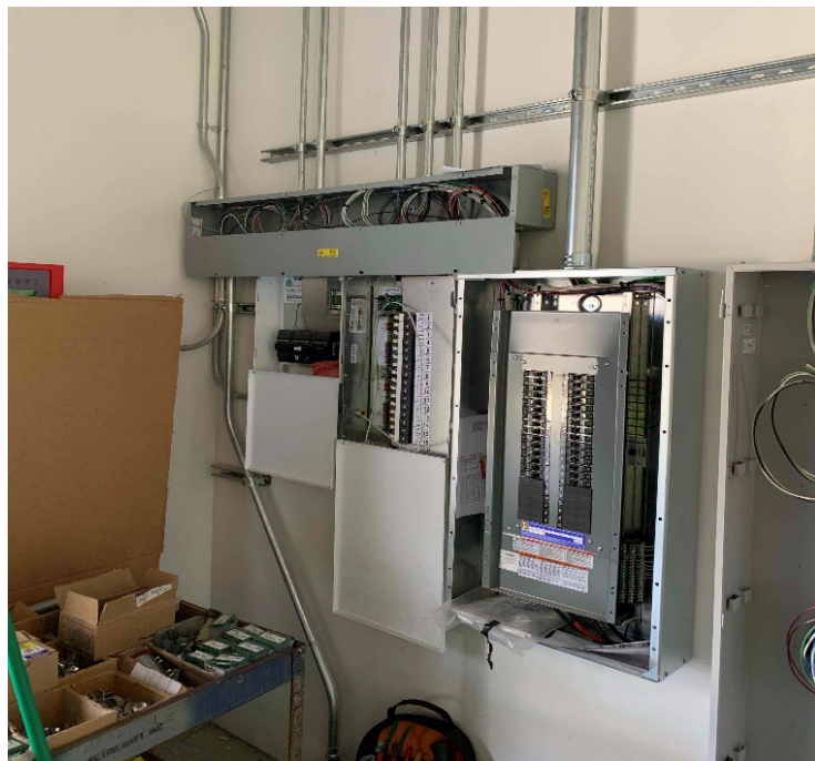
Electrical Controls and Breaker Installation Progress
