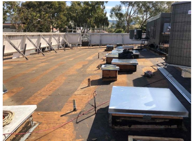
Building 2200 Roof Demo
