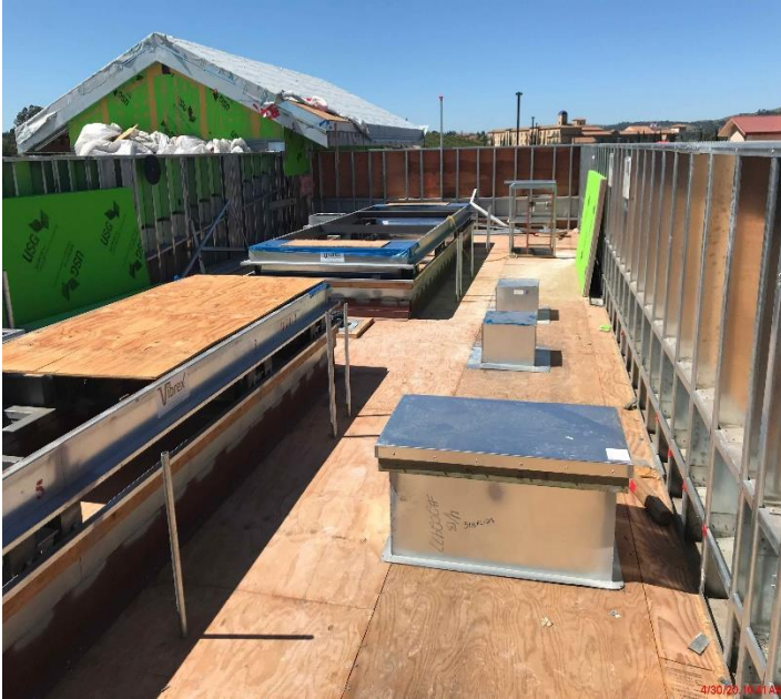
HVAC Equipment Curb Installation Progress
