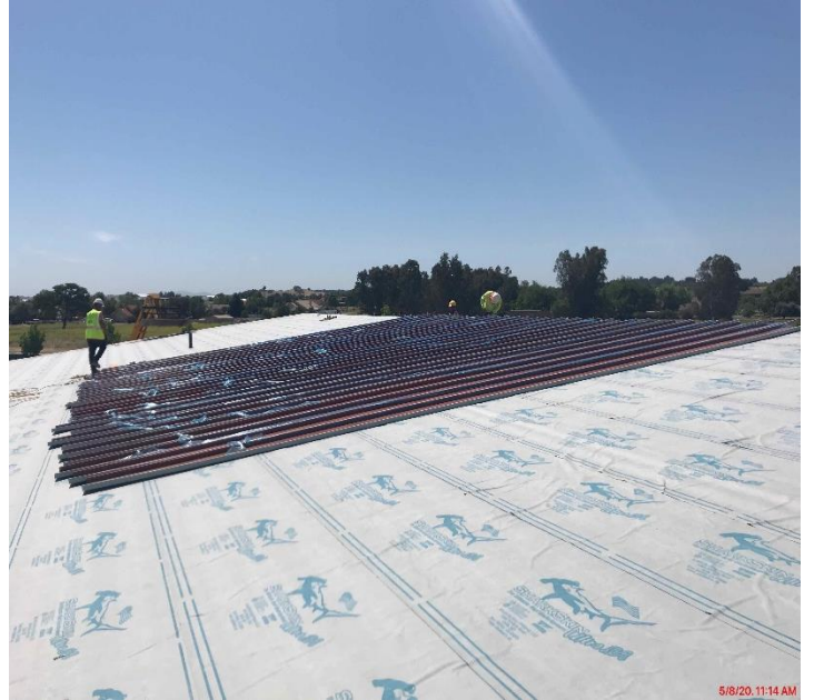
Installation of Standing Seam Metal Roof
