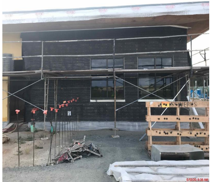
Start of Lath and Plaster Installation
