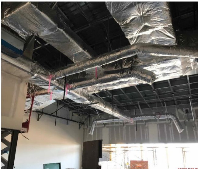
HVAC Duct Insulation Progress
