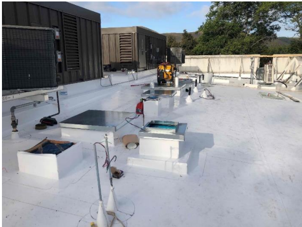
New Roof Insulation/Membrane Installed
