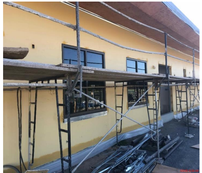
Exterior Window Frame Installation
