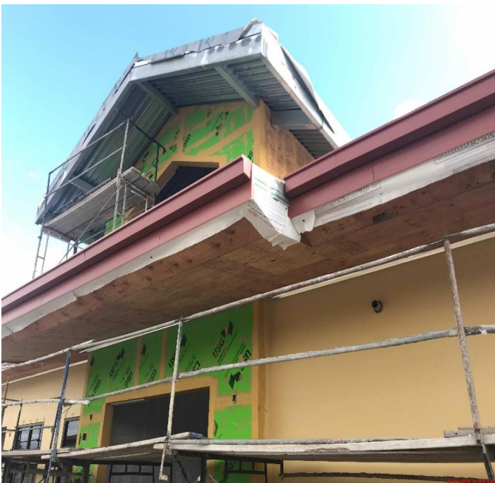
Gutter Installation at Main Entry
