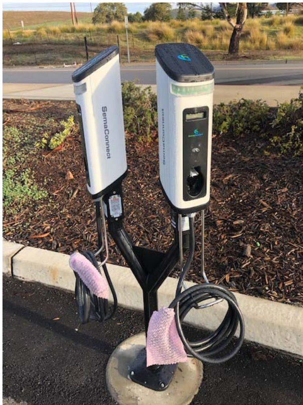
EV Charging Stations
