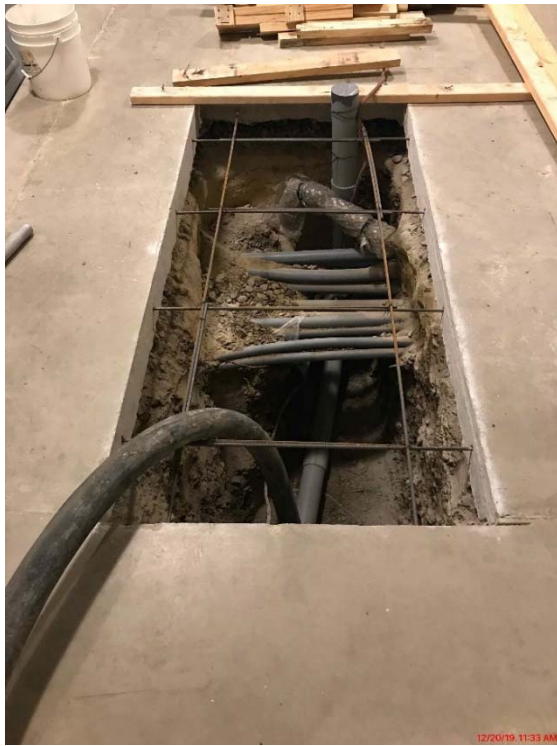
New Cabling into Electrical Room
