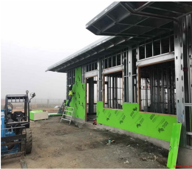
Exterior Sheathing Progress
