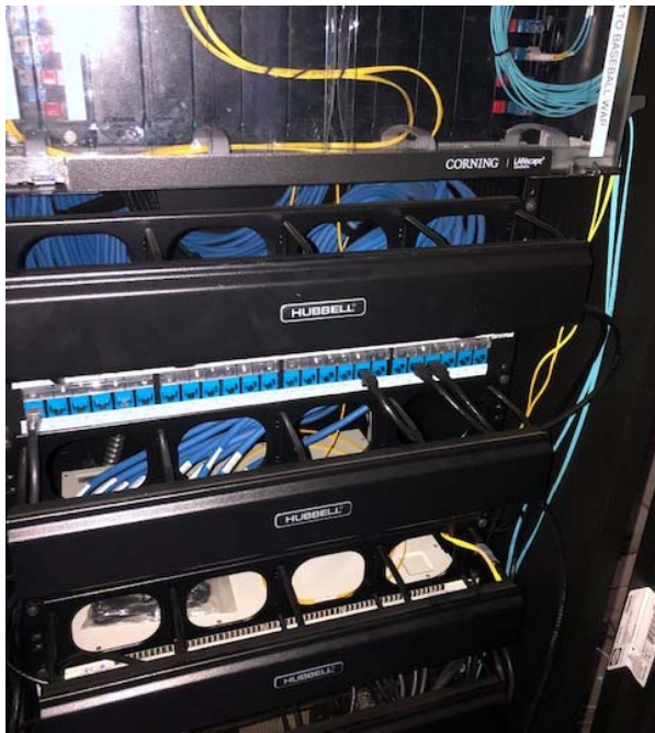
New Fiber Runs and Terminations
