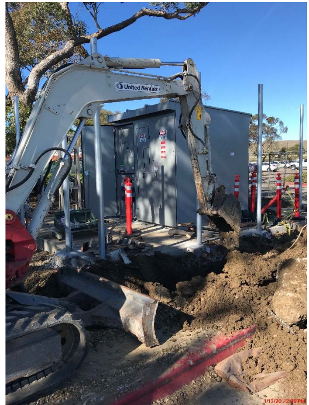
New Switchgear Installation
