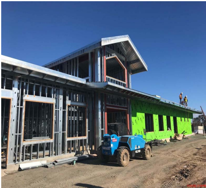
Front Entry Framing and Sheathing Progress
