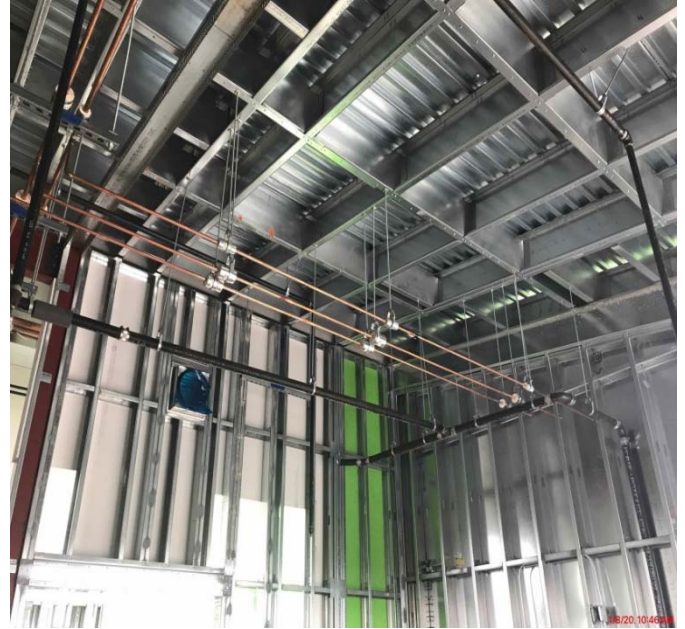
Installation of HVAC Hangers and Piping
