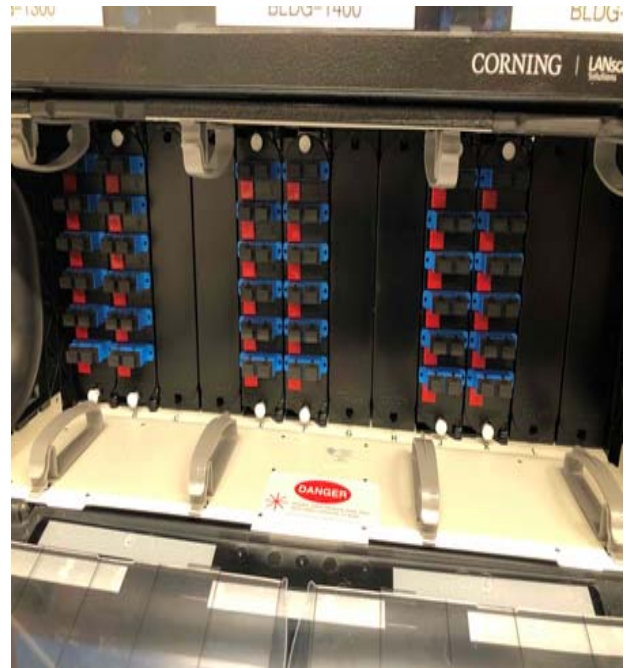
New Fiber Runs and Terminations
