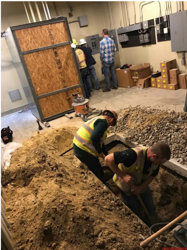
Trenching for Cable Pathways
