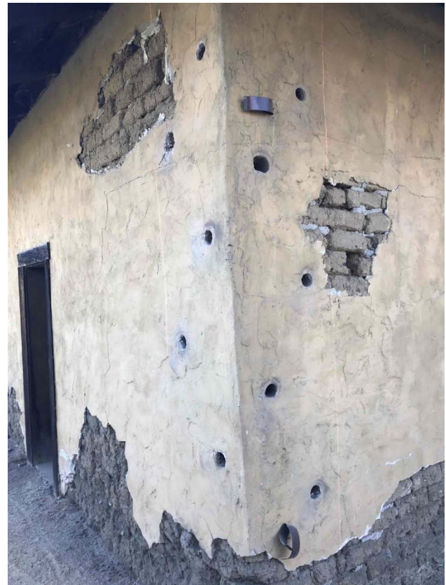
Core Drilling for Fiberglass Rods
