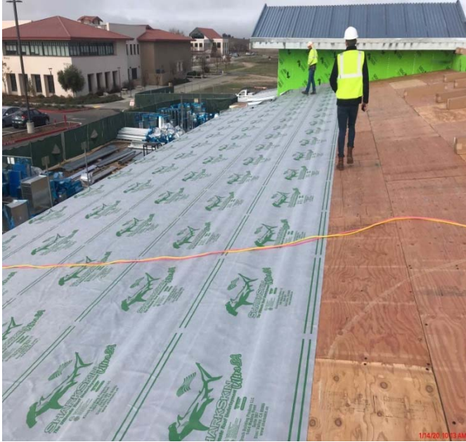
Roof Dry-in Progress
