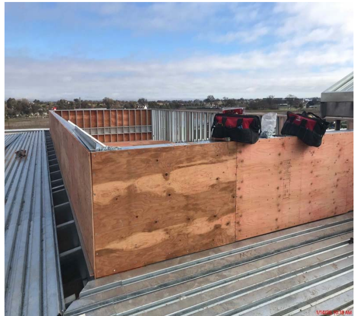
Parapet Well Progress
