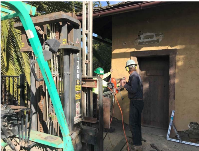
Core Drilling for Fiberglass Rods
