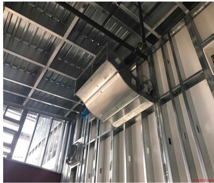
Ductwork Installation Progress
