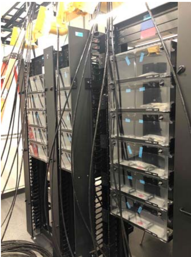
Fiber Runs terminated in the new Data Center
