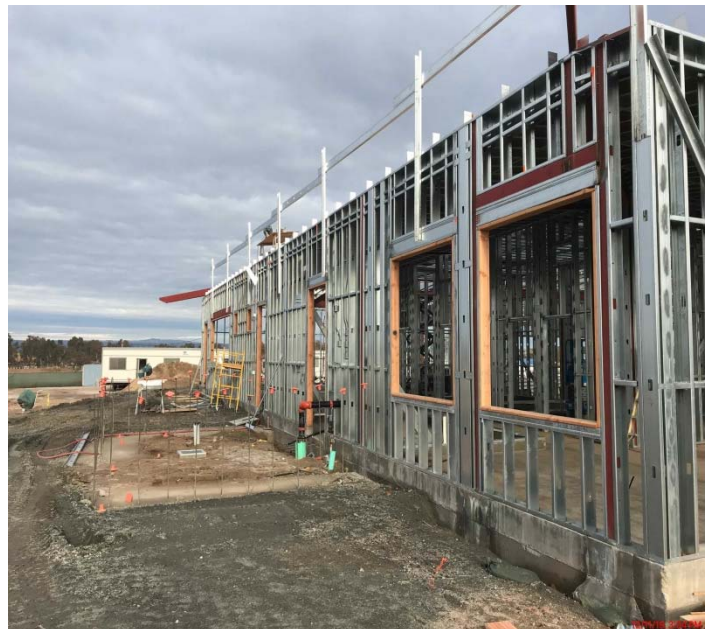
Wood Nailer Installation Complete
