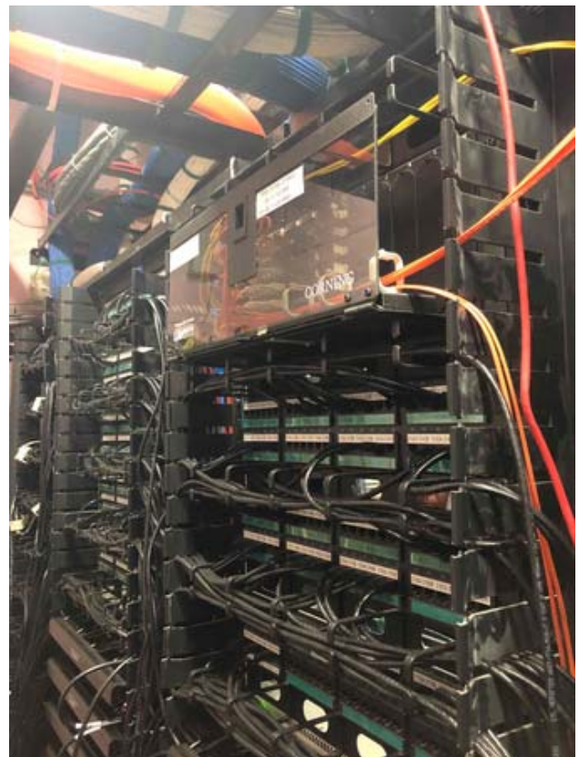
Fiber Runs terminated in the new Data Center
