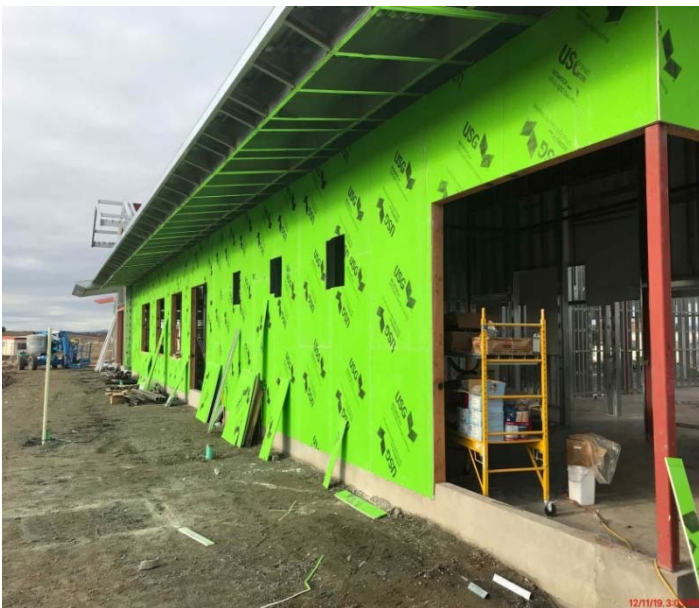
Exterior Sheathing Progress
