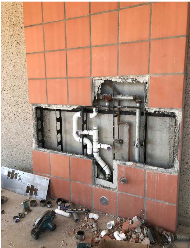
New Drinking Fountain & Hydration Station Installation
