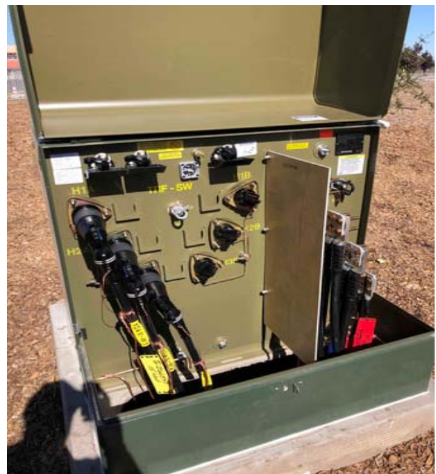
New Transformer on SLO Campus
