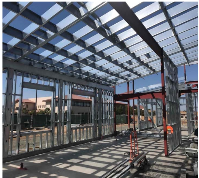
ECE Building Metal Framing Progress
