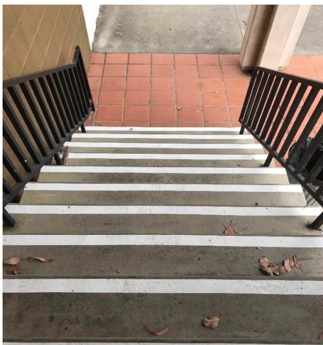
Contrasting Strip at Building 2400 Stairs
