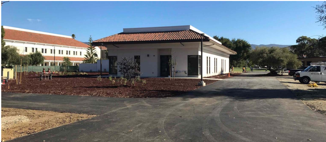
Data Center Exterior with New Landscaping and Asphalt Paving
