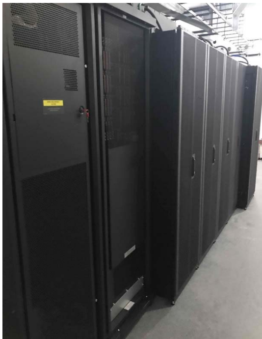
New Equipment in the Machine Room
