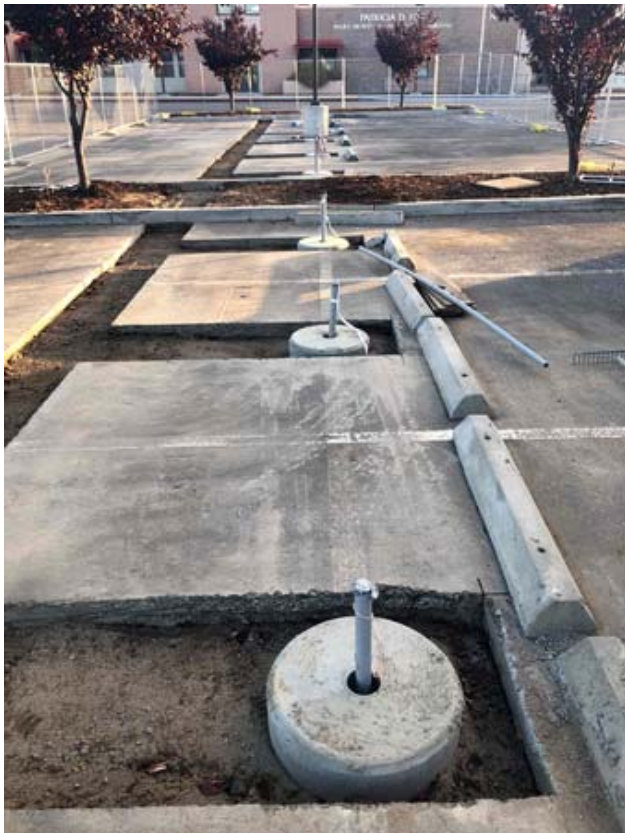
Bases for New Charger Stations in North County
