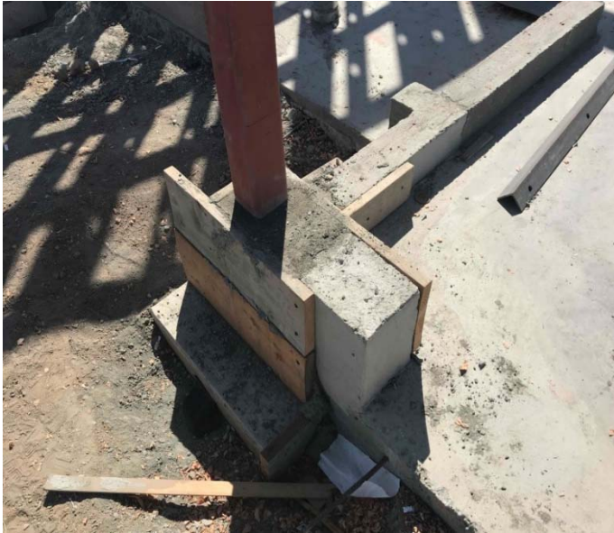
Placement of Column Block outs
