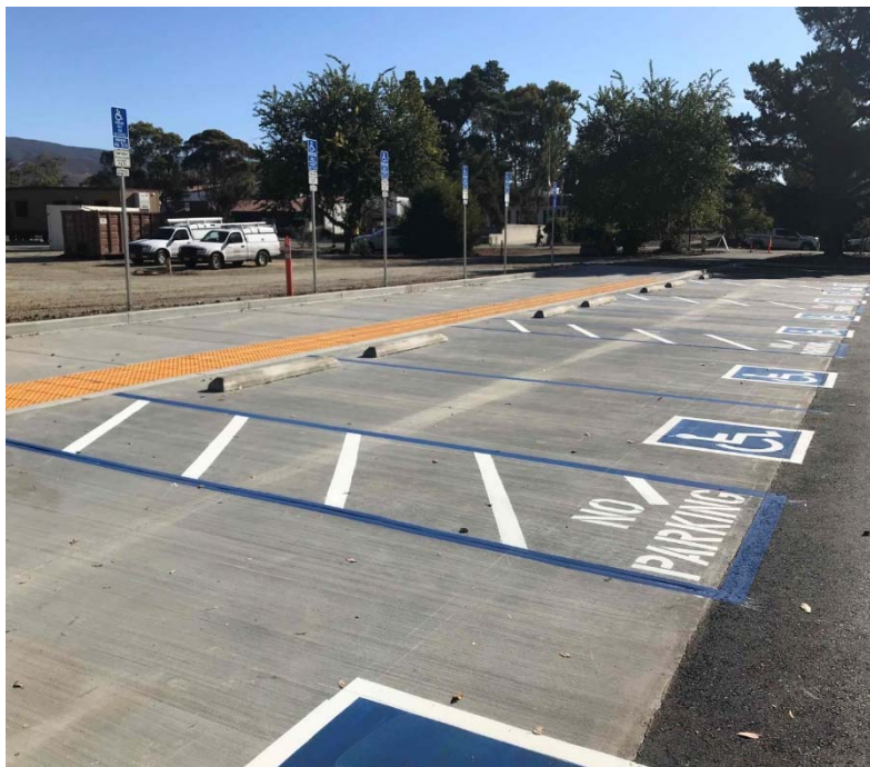
New ADA Parking Stalls in Lot 5
