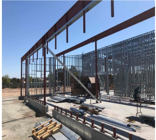
Structural Steel Installation Nearing Completion
