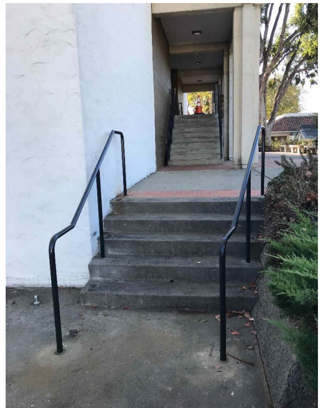
Handrail installation at Building 2400
