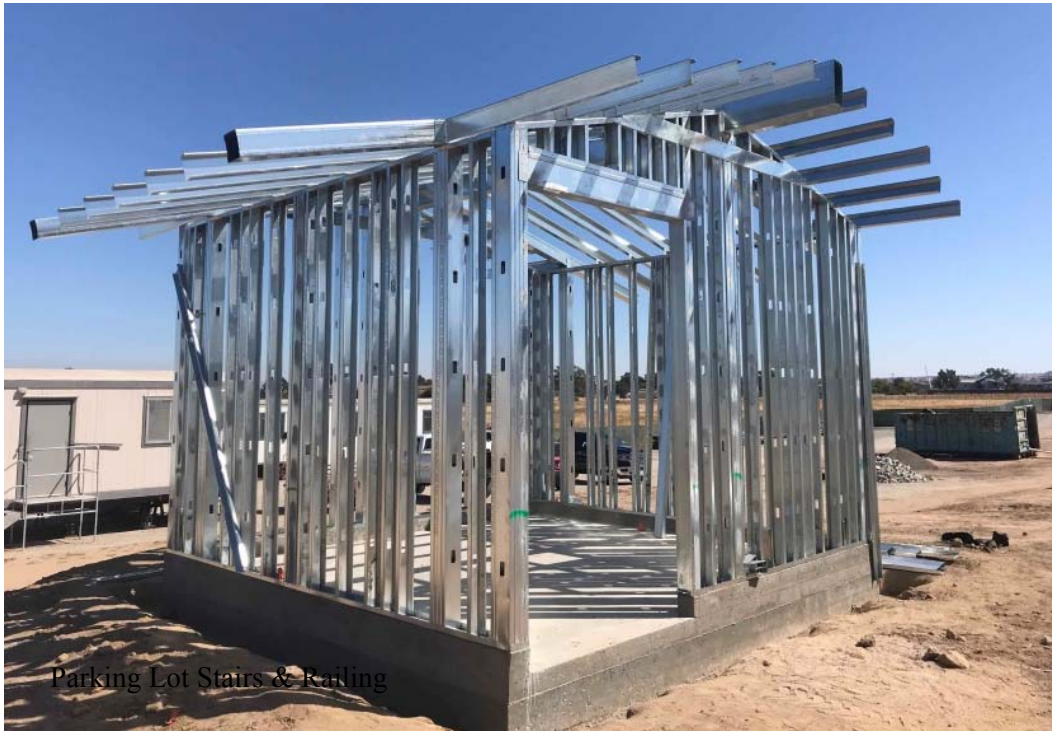
Framing Progress on the Exterior Storage Buildings
