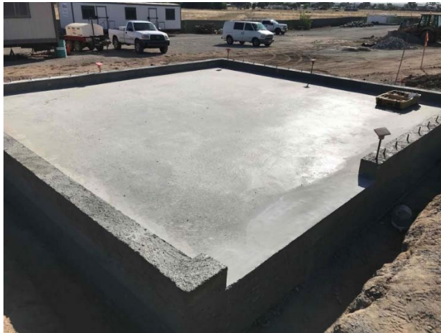
New Storage Building Slab & Curbs
