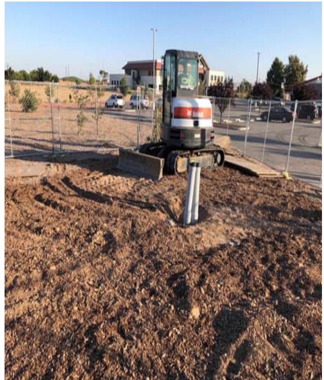
Trenching and Conduit Installations
