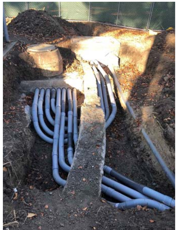
New Underground Conduits into Existing Vaults
