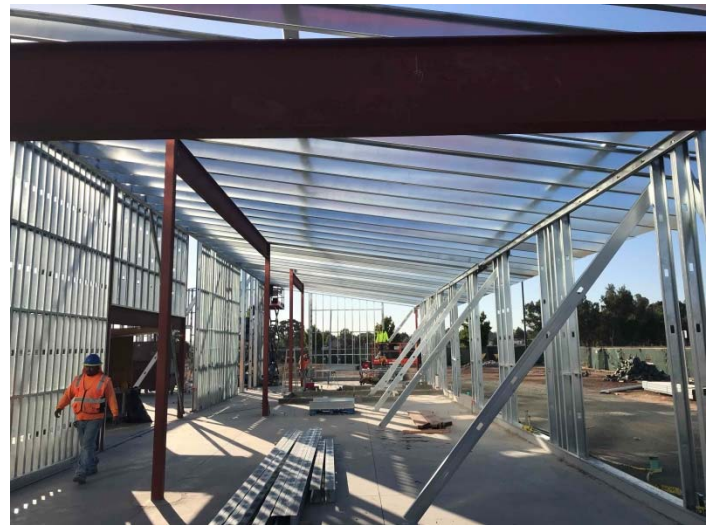
Metal Framing at ECE Building
