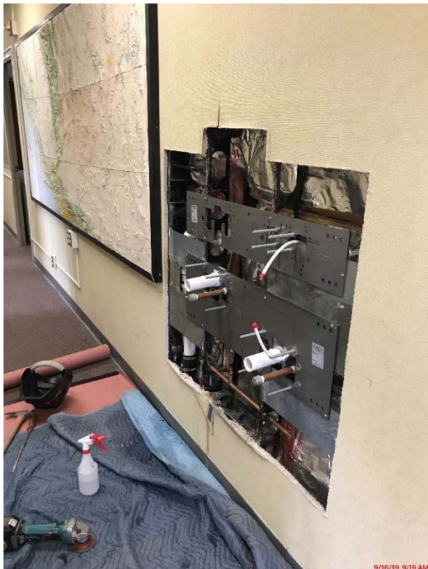
New Drinking Fountain Installation
