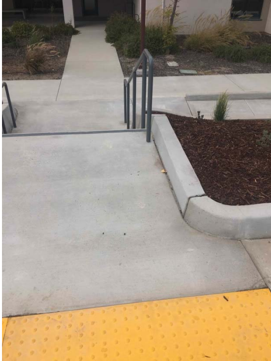
Parking Lot Stairs & Railing
