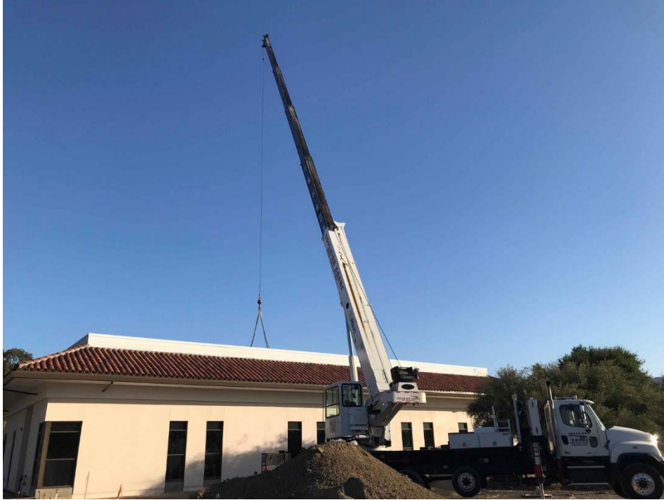
Crane Installation of HVAC Units on the Roof.
