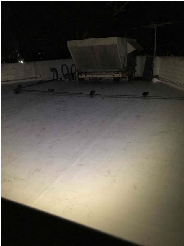
New Roofing at Building 2400
