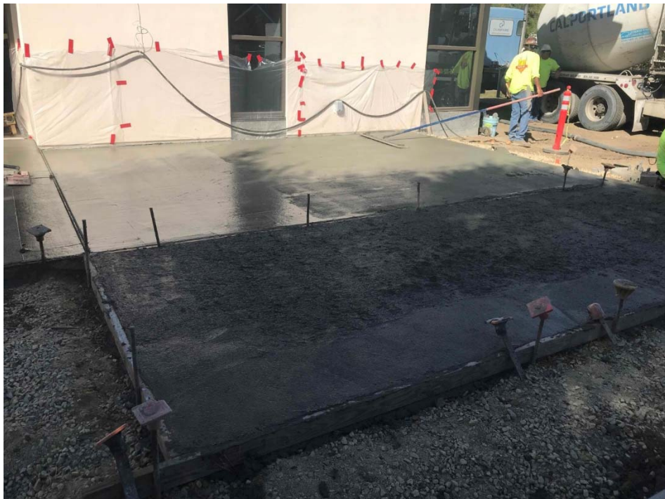
Exterior Concrete Flatwork Installation
