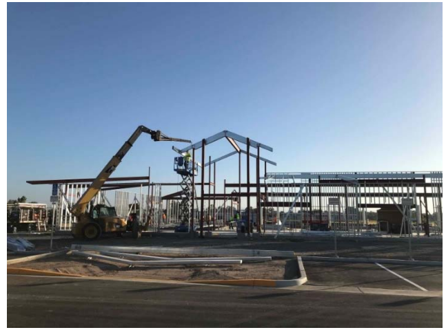
Exterior High Roof Framing
