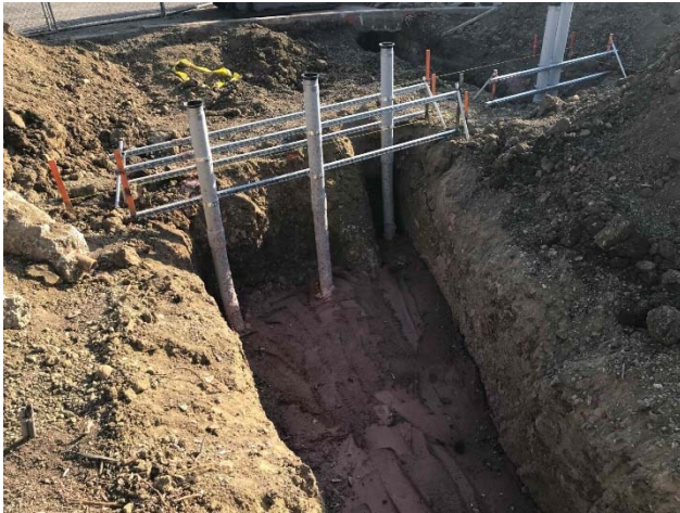
New Conduit and Slurry Installation
