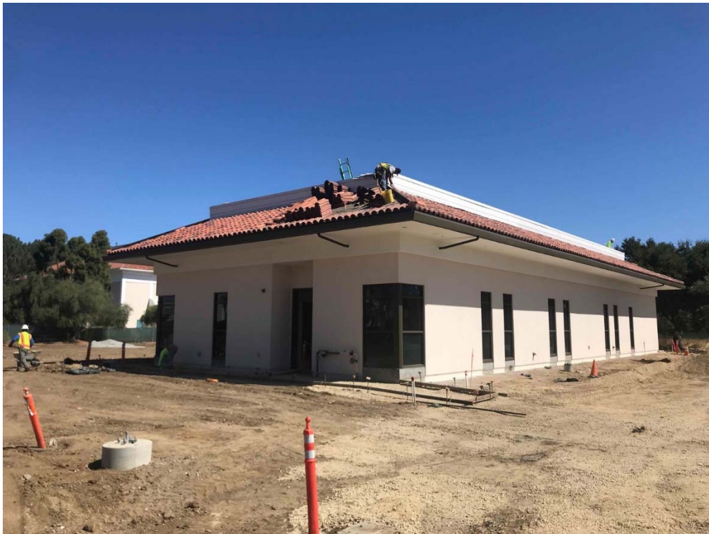
Data Center Exterior – Plaster, Windows, Roof Tile, Rough Grading
