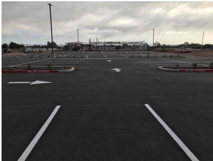
New Parking Lot Complete
