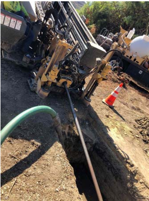
Directional Boring for New Conduit Installation
