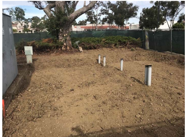
Conduit Install at New Equipment Pad Location
