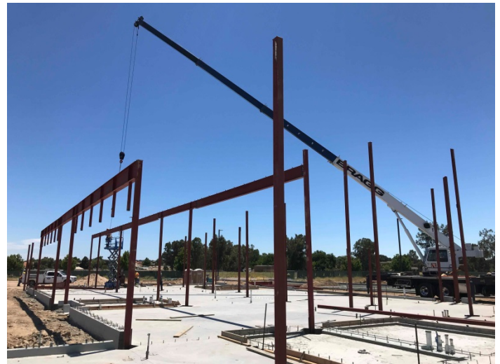
Steel Erection
