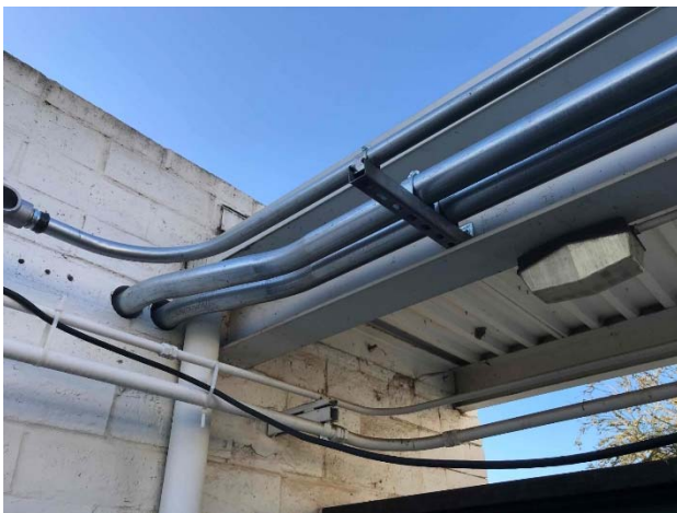
Electrical Conduit for Backup Generator to the Chiller Yard
