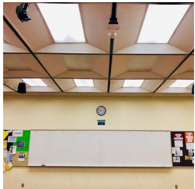
New ceiling mounted WAP Installed in Building 1100
