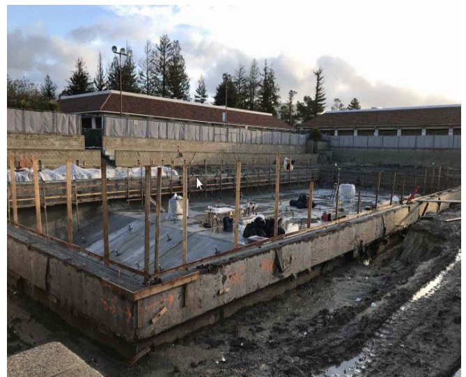
Backfill around the Competition Pool
