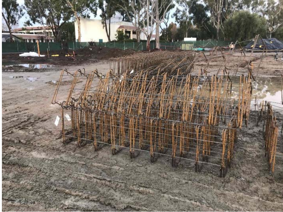
Grade Beam Rebar Ready to Install
