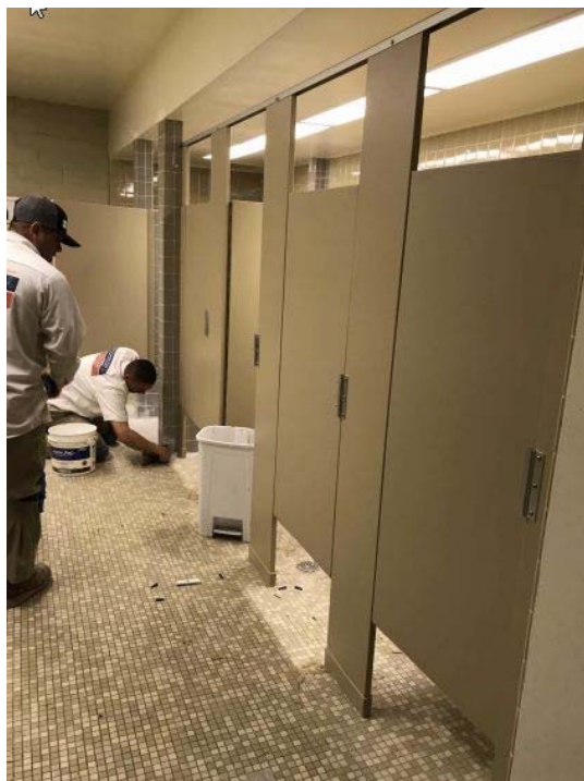
Building 1400 Restroom Partitions Installed
