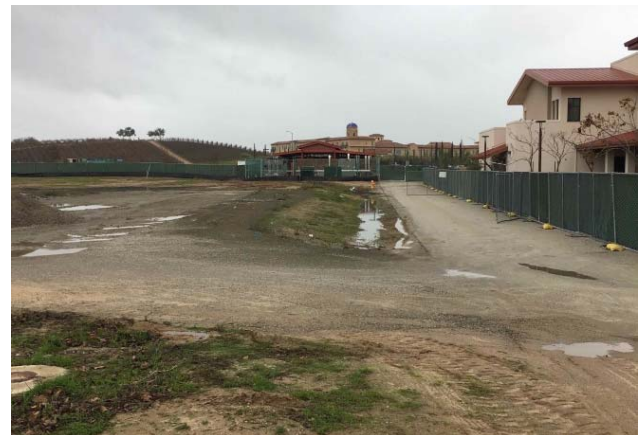
Installation of Temp Fencing and BMPs
