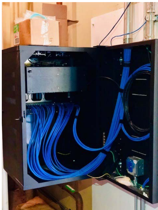
Termination in New Rack
