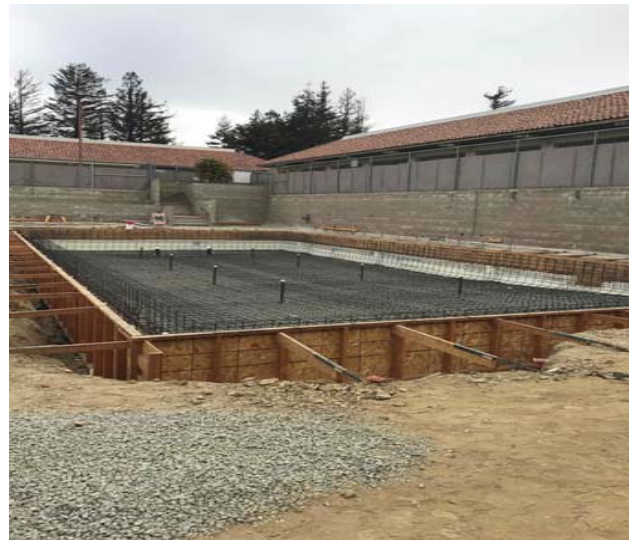
Teaching Pool Formwork & Reinforcement progress
