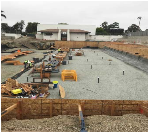
Competition Pool Formwork & Recirculation piping
