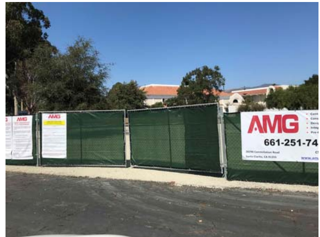
Data Center Construction Site Entrance
