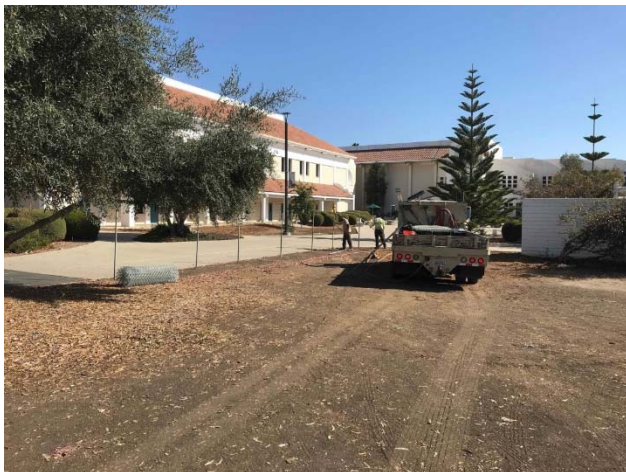
Installation of Temporary Fencing
