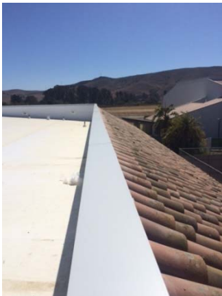
Building 1000 Parapet Cap
