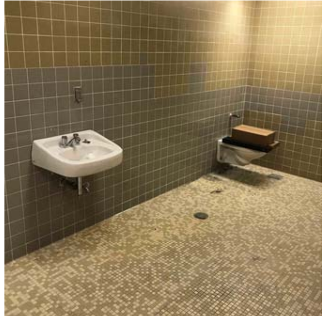
Building 1300 Fixture Installation
