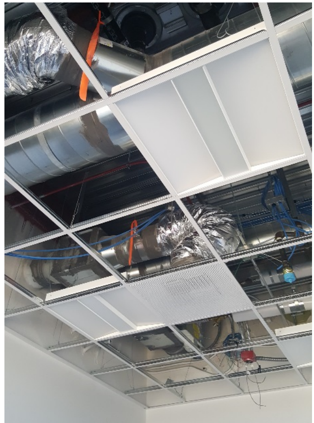
Ceiling Grid, Light Fixture and Diffuser Installation
