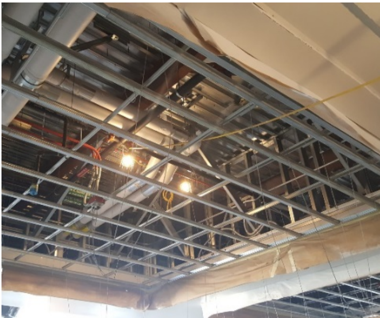
Acoustical Plaster Ceilings Underway
