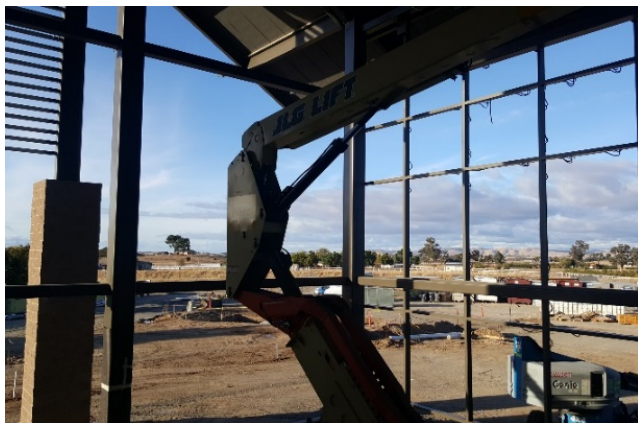
Curtainwall Installation in Progress at Main Entry
