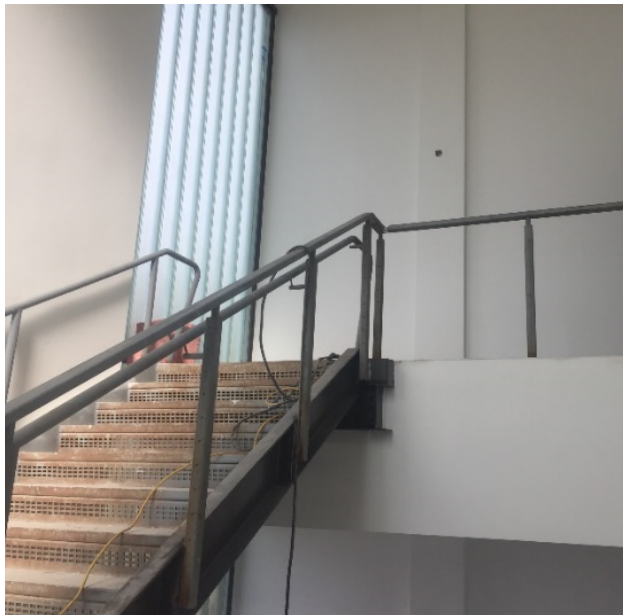
Interior Stair Handrail Installation
