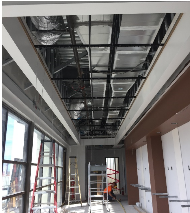
Metal Ceiling Grid Installation at Second Floor
