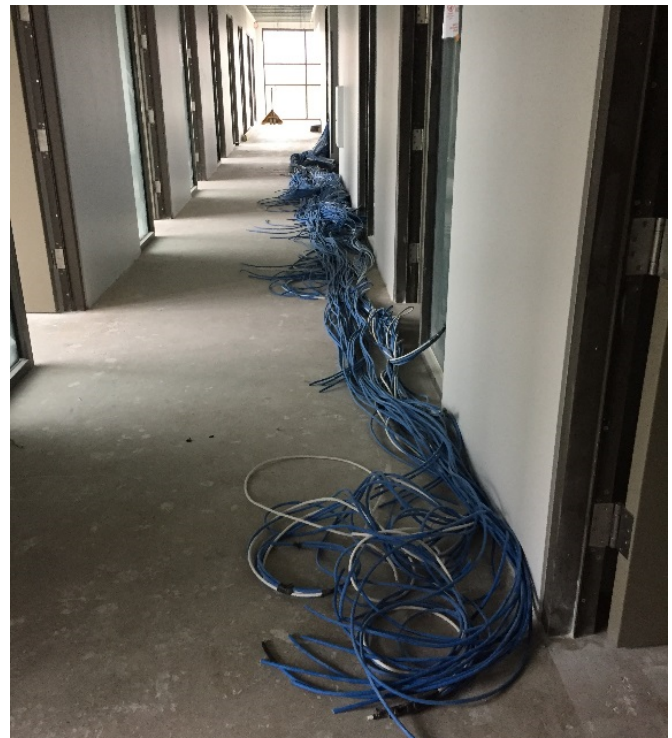
Second Floor Data Cable Pull
