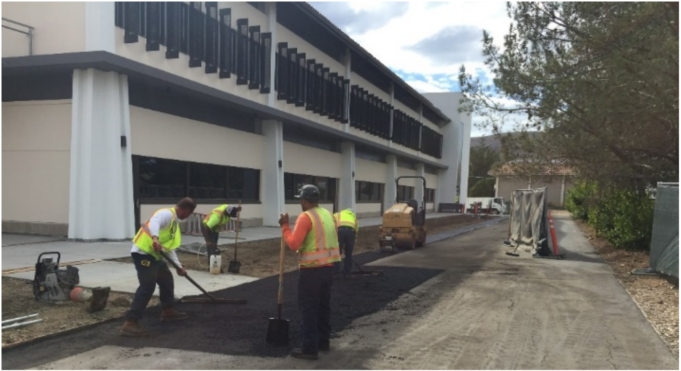
Asphalt Concrete Placement along West Side of Building
