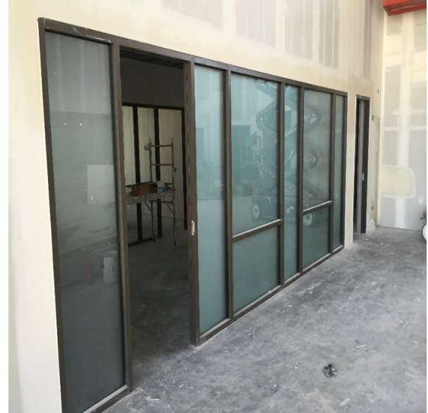
Second Floor Storefront Windows
