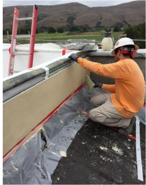
Roof Parapet Plaster
