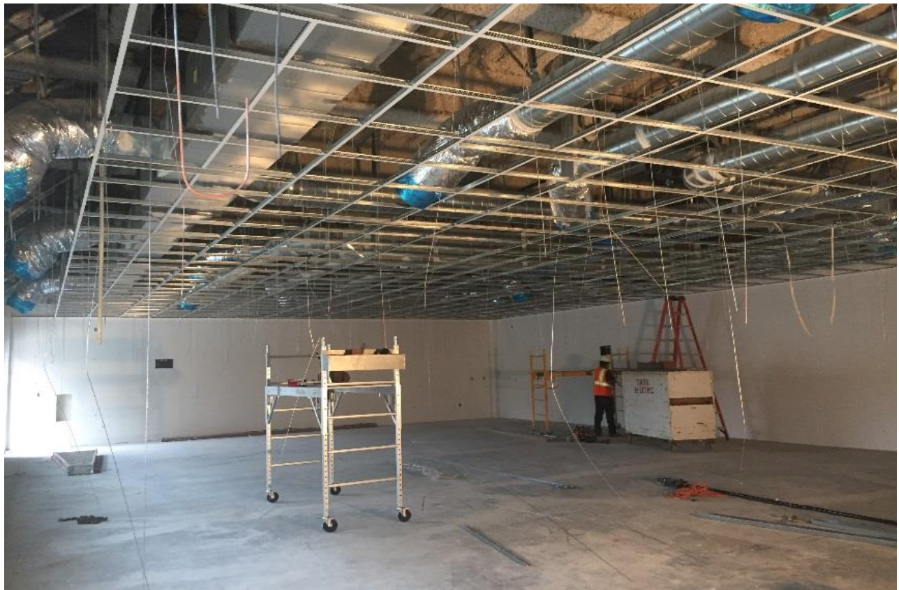
Ceiling Grid Installation
