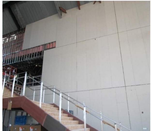
Entry Lobby, Insulation and Drywall
