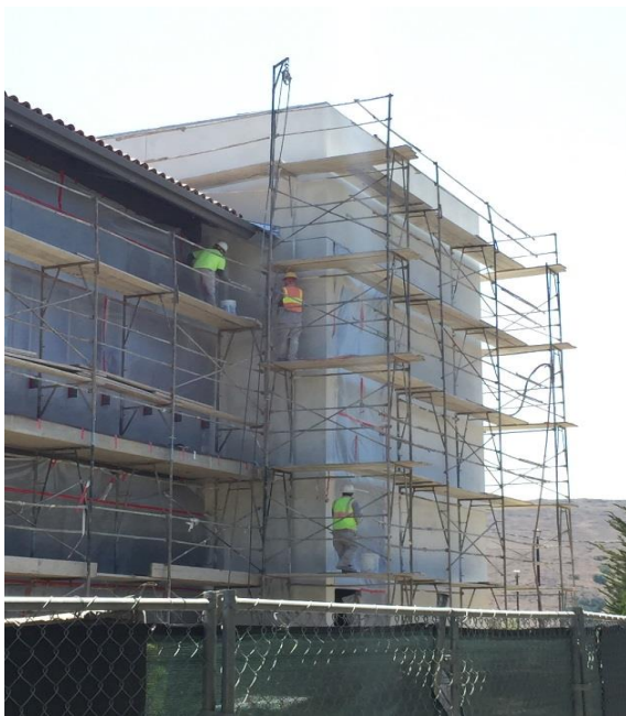
Stair Tower Plaster in Progress
