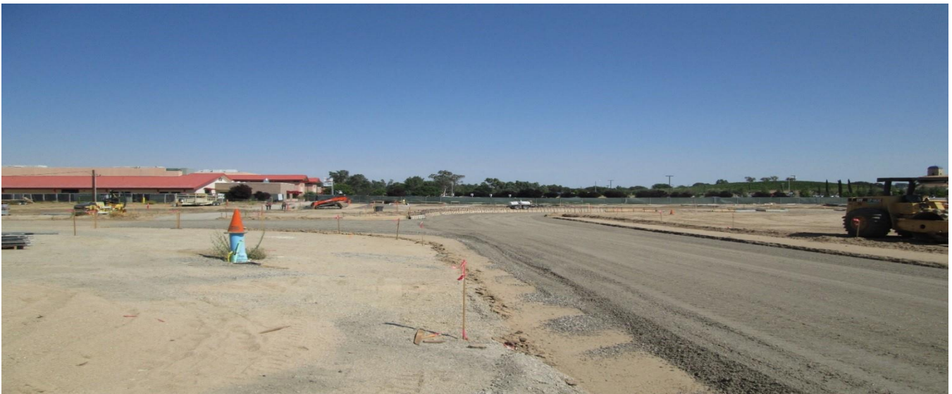
New Roadway Connecting Parking Lot 10 and 11
