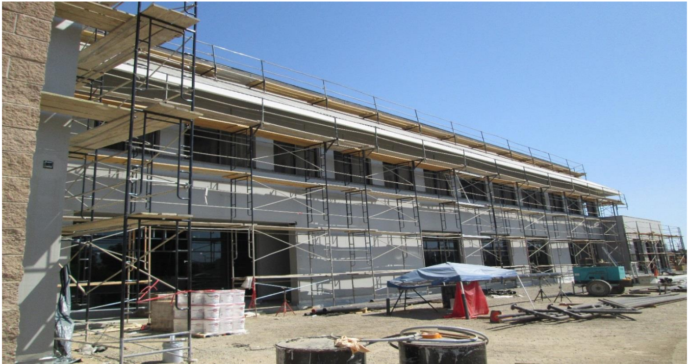
Exterior with Storefront Windows Installed
