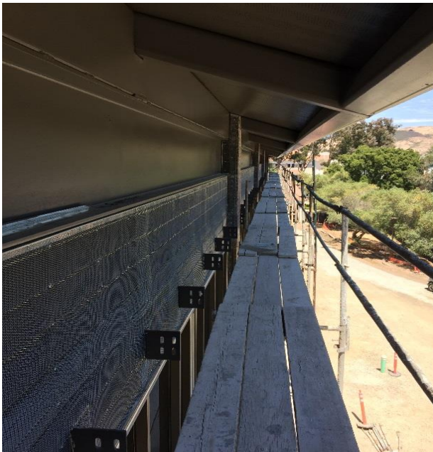
Installation of Metal Lath
