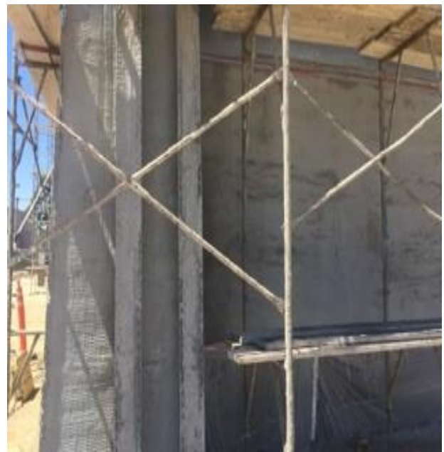
Plaster Installation Progress
