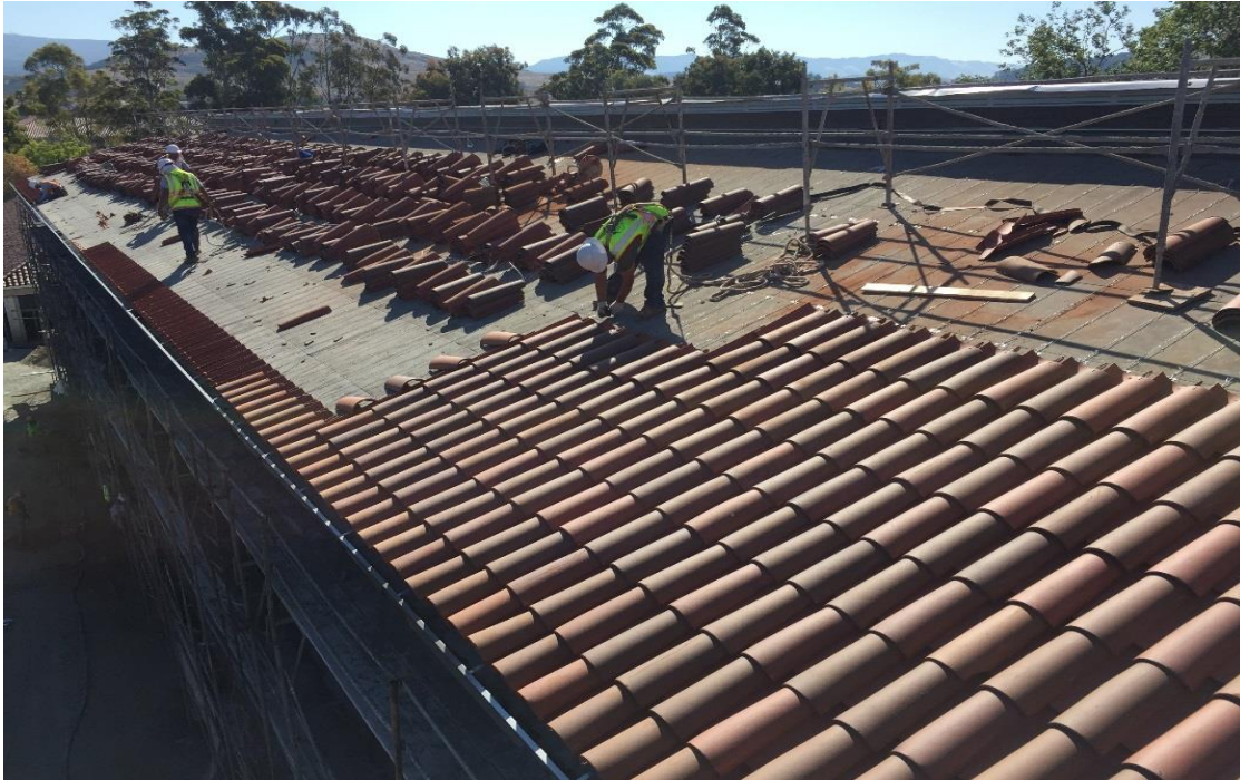
Roof Tile Installation
