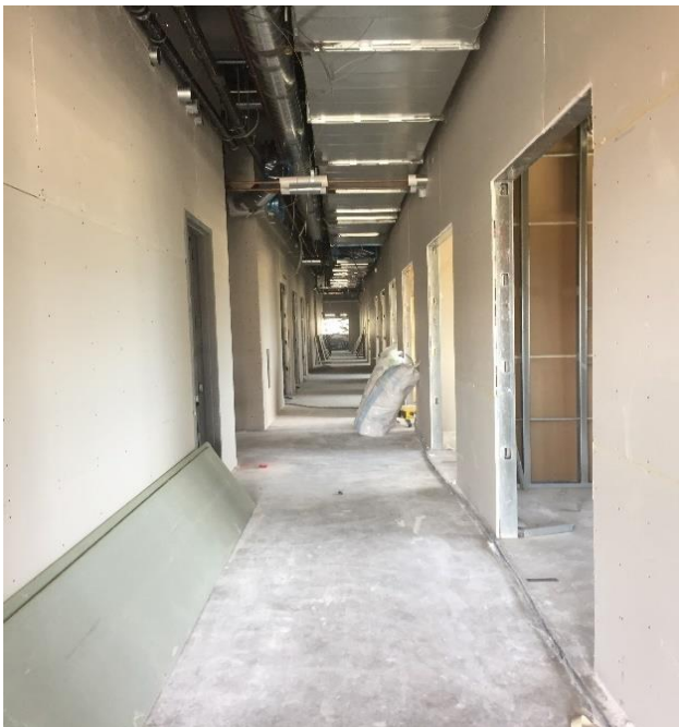
Second Floor Corridor Wall Progress
