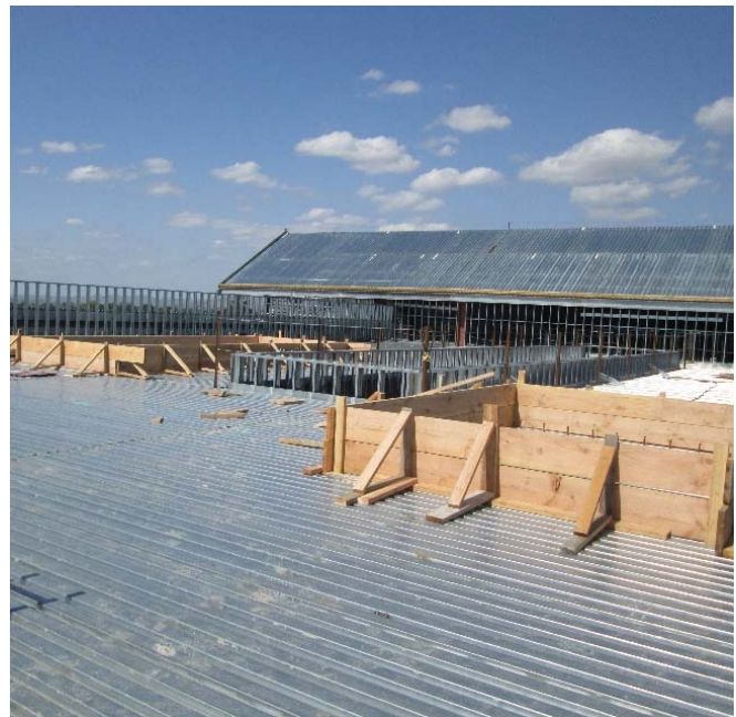
Forms for Rooftop Concrete Pads
