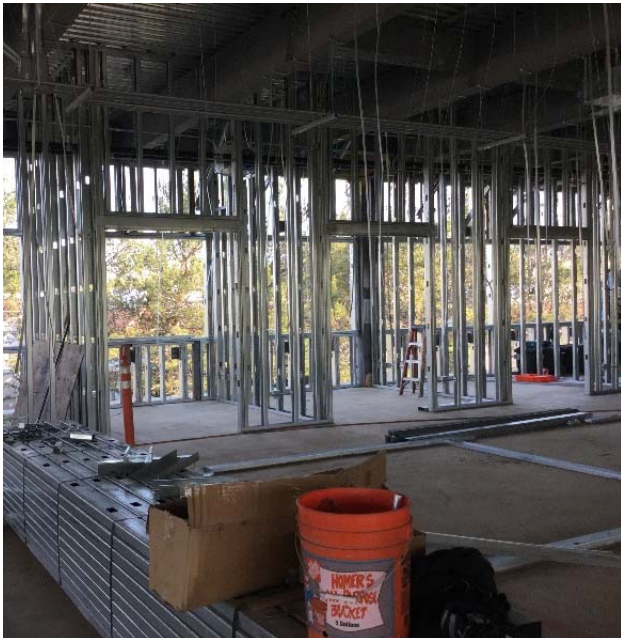
Second Floor Office Framing Progress
