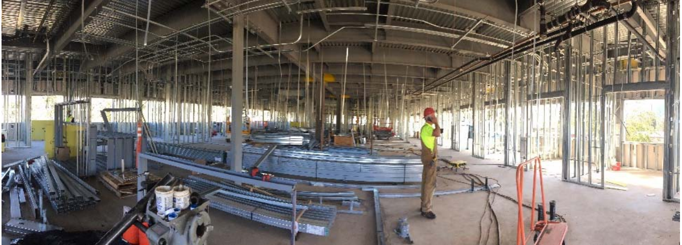
Second Floor Progress
