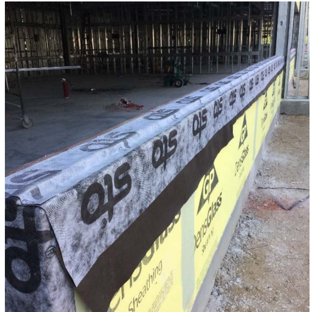
Installation of Waterproofing around Windows
