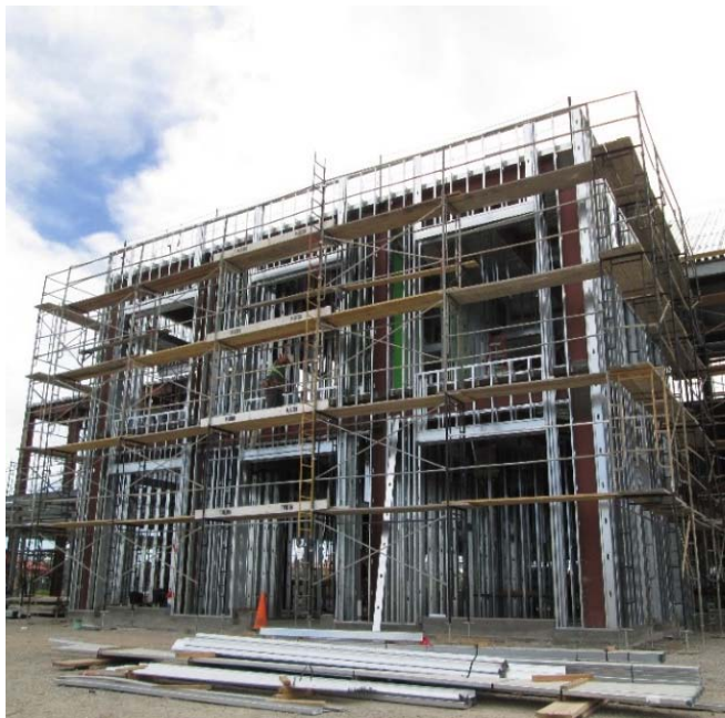
Scaffolding and Exterior Wall Framing
