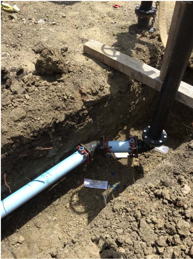
Building's Fire Water Line Connection
