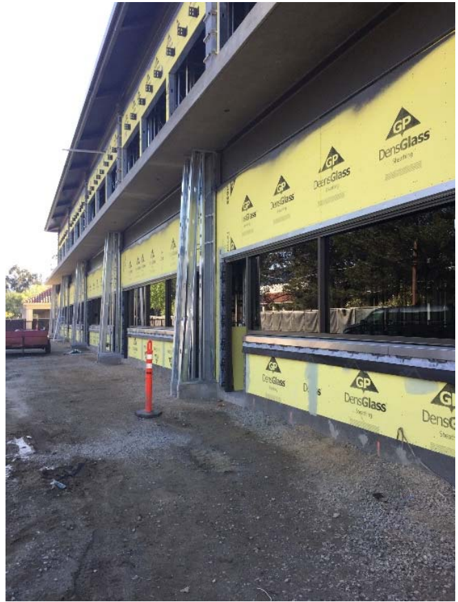
Exterior Sheathing and Window Install Progress
