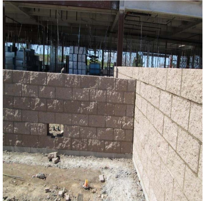
Concrete Masonry Walls
