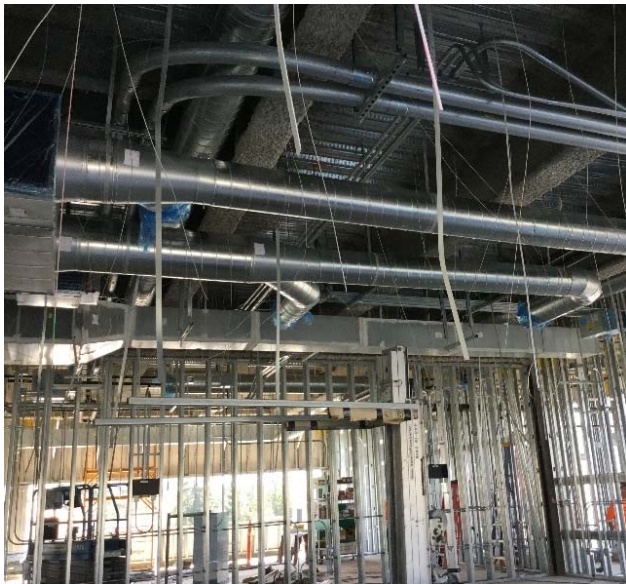
First Floor MEP Component Installation
