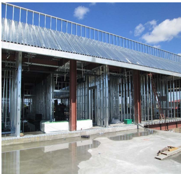
Interior Wall Framing
