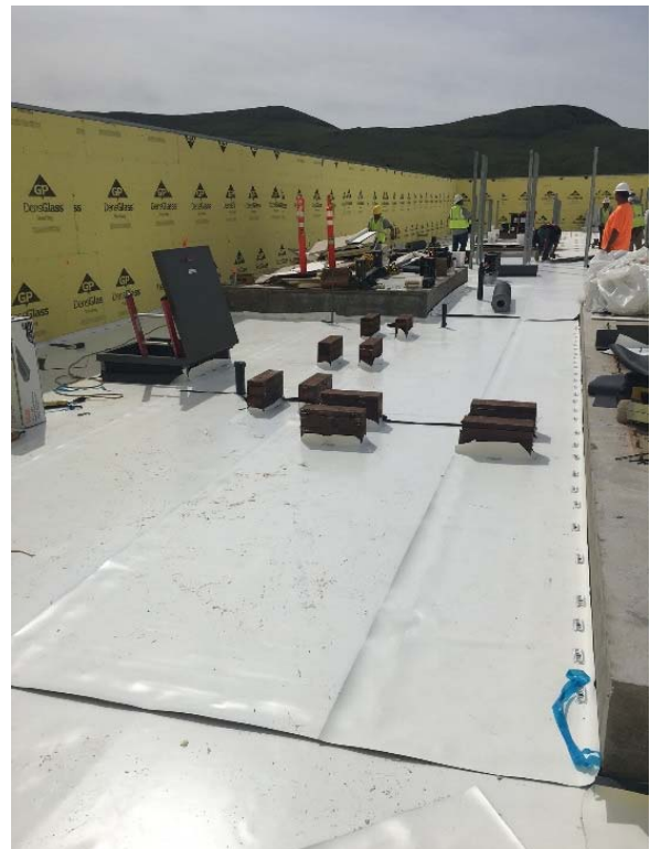
Single Ply Roofing Installation
