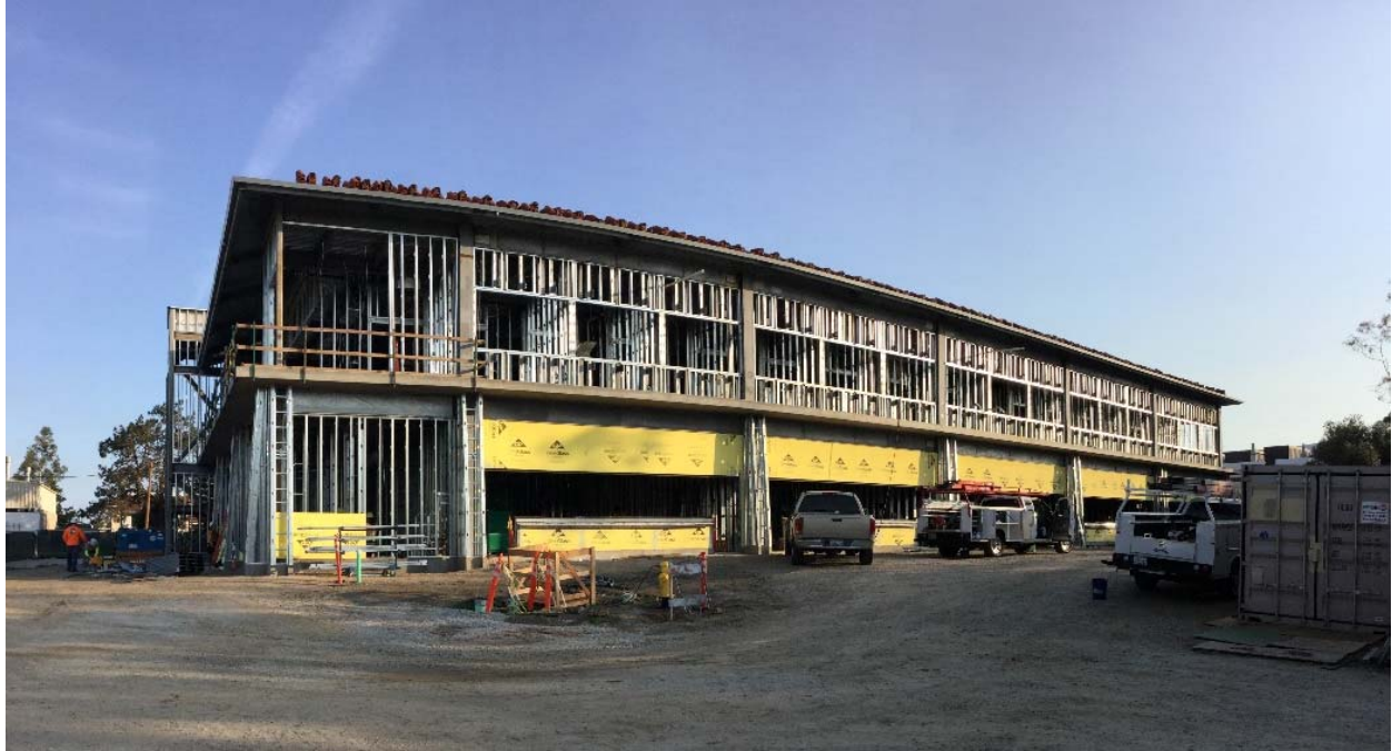
Framing and Sheathing Progress on the Southside of the Building
