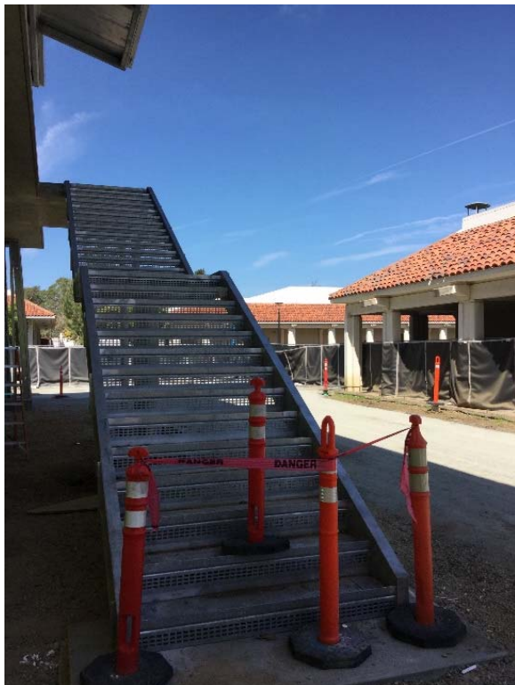
Installation of the Exterior Stairs
