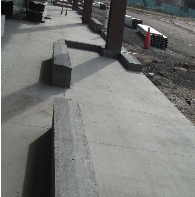
Completed Perimeter Curbs
