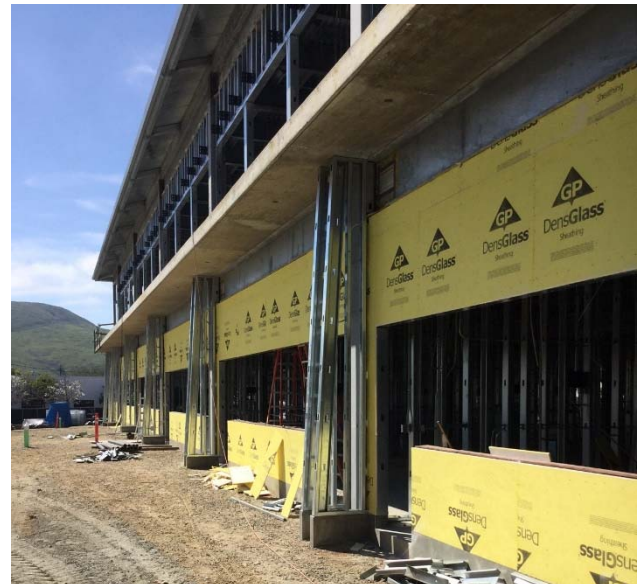
Sheathing at Exterior Walls
