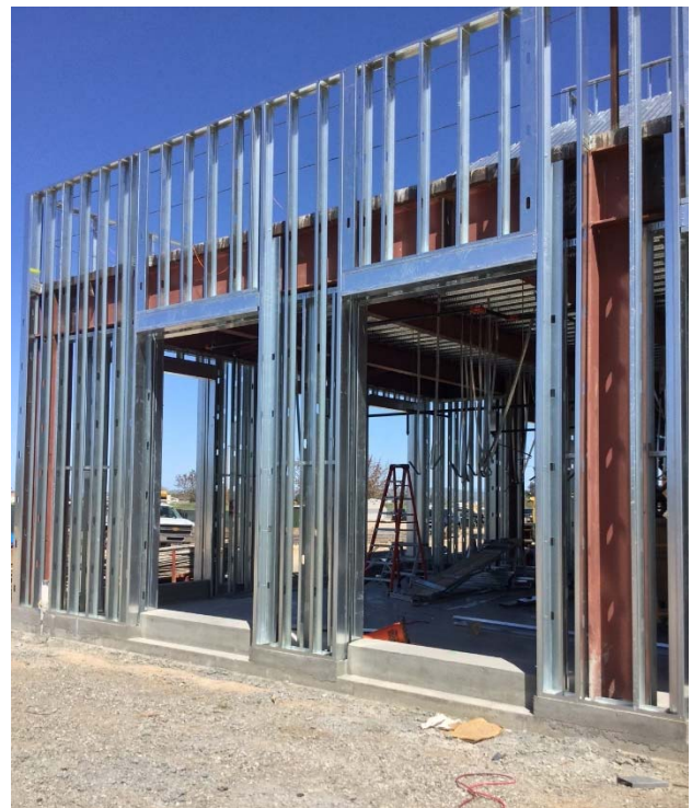
Exterior Wall Framing
