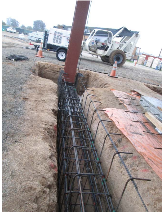
Grade Beam Reinforcing Steel
