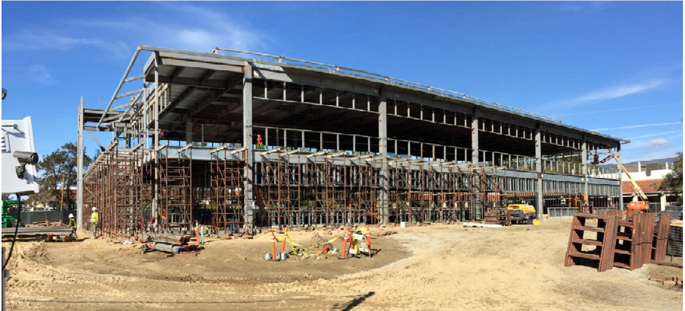
Installation of Shoring for Cantilever Deck
