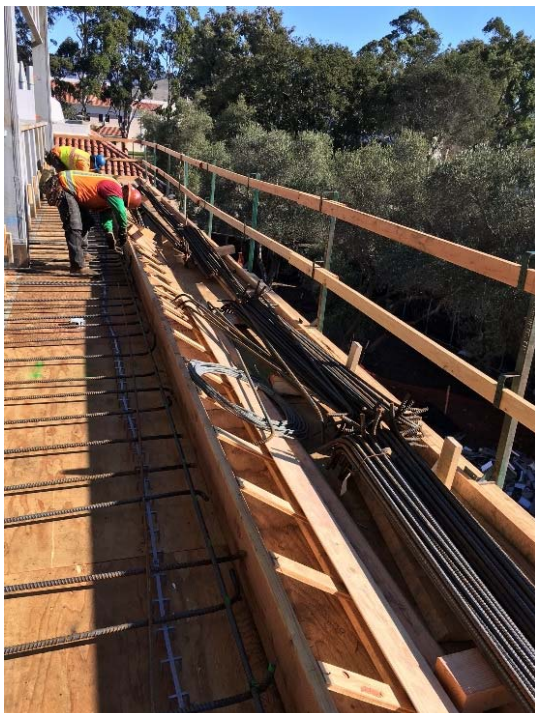
Installation of Plywood and Rebar at the Cantilevered Deck
