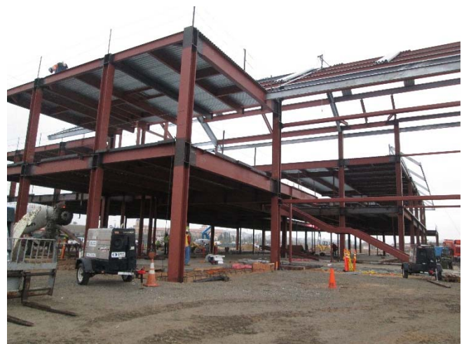
Roof Decking Installation
