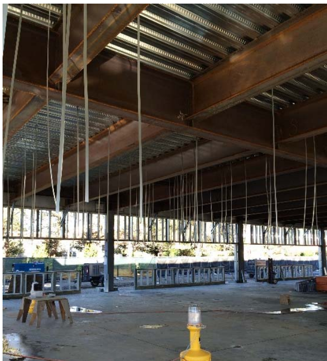
Deck Insert Installation
