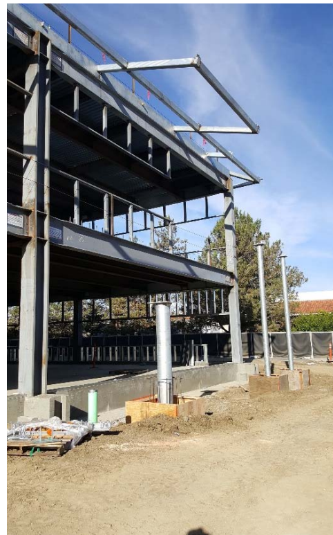
Placement of Columns for Exterior Stairs
