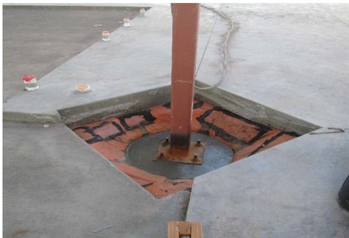
Grouting Column Bases
