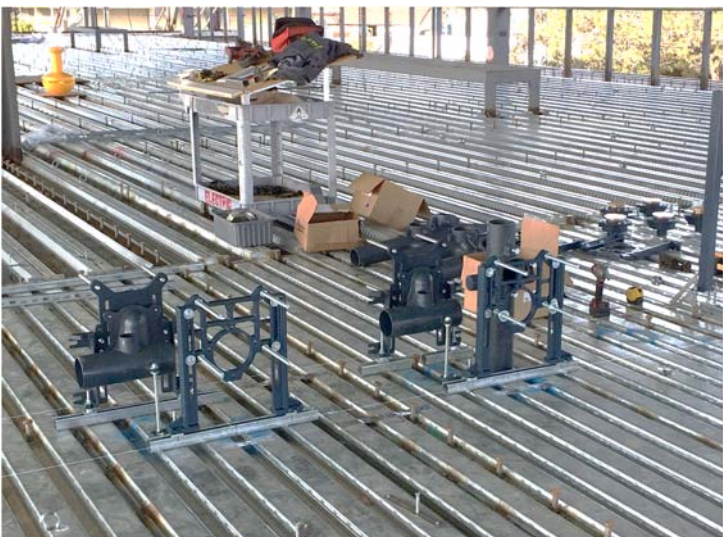
Rough Plumbing on the Second Floor
