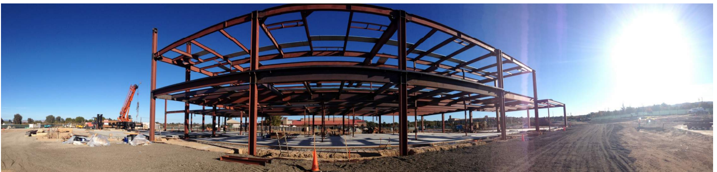
Structural Steel Erection Continued
