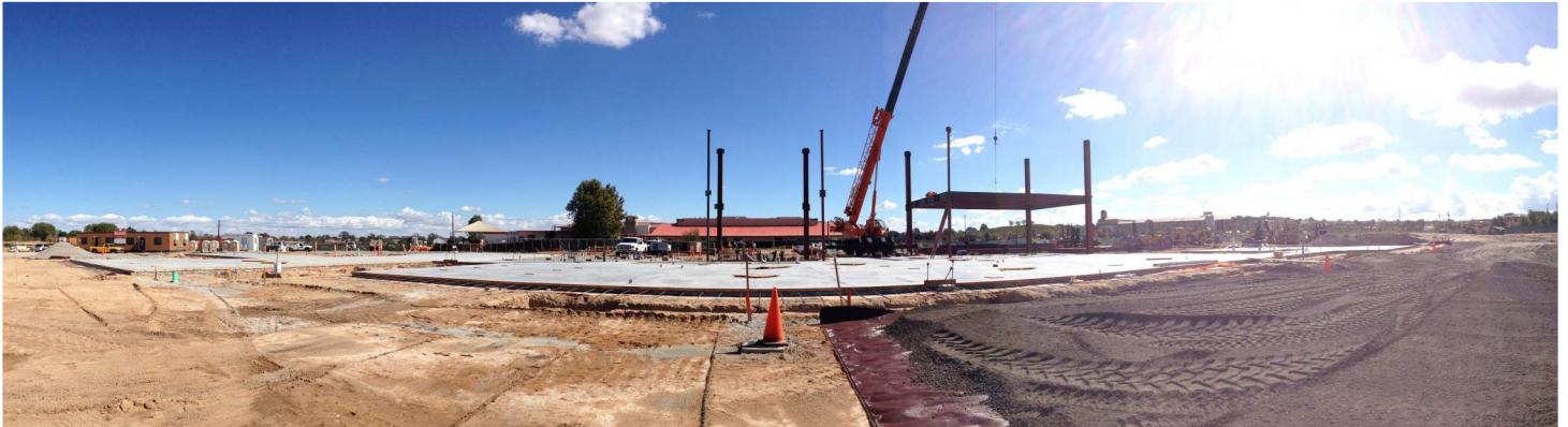
Start of Structural Steel Erection
