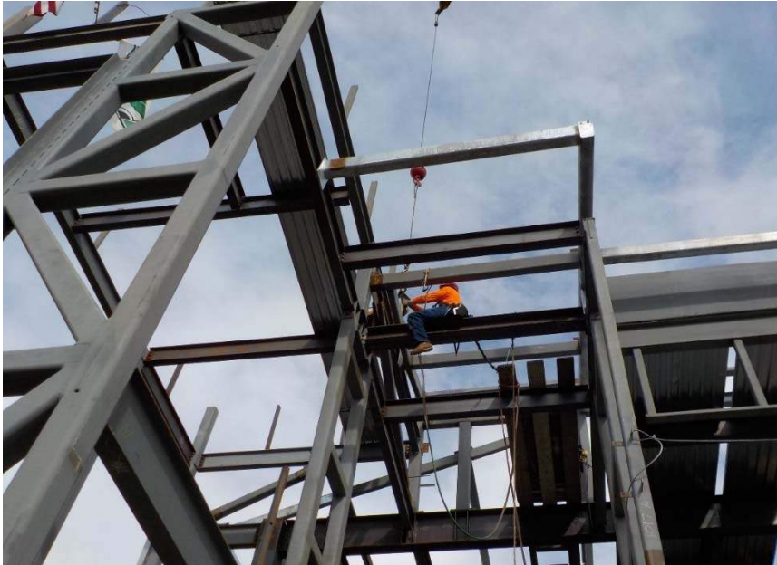
Installation of Steel Near the Elevator Hoistway
