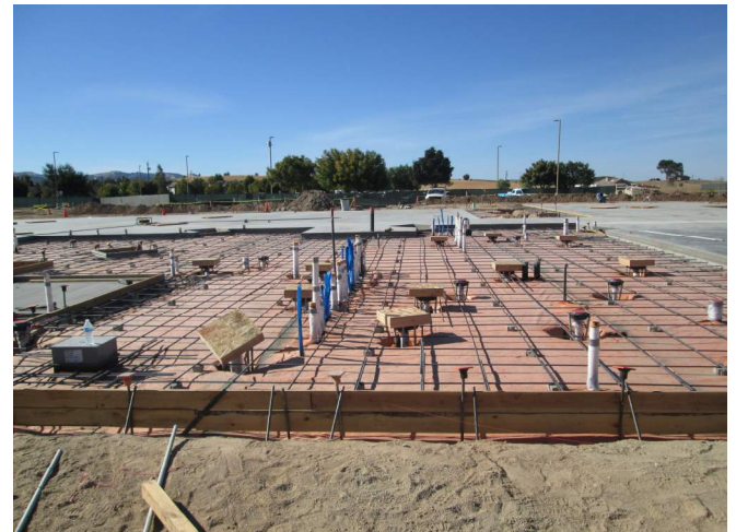
Depressed Slab Area
