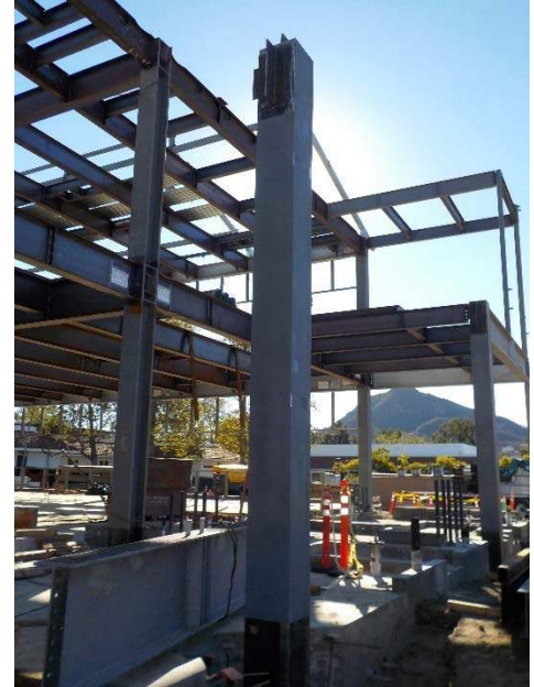
Built-up Box Column at West End of Building
