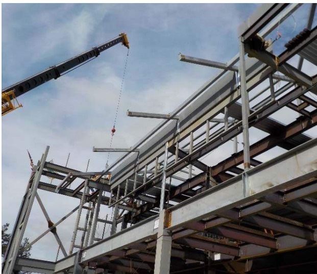
Structural Steel Erection at West End of Building
