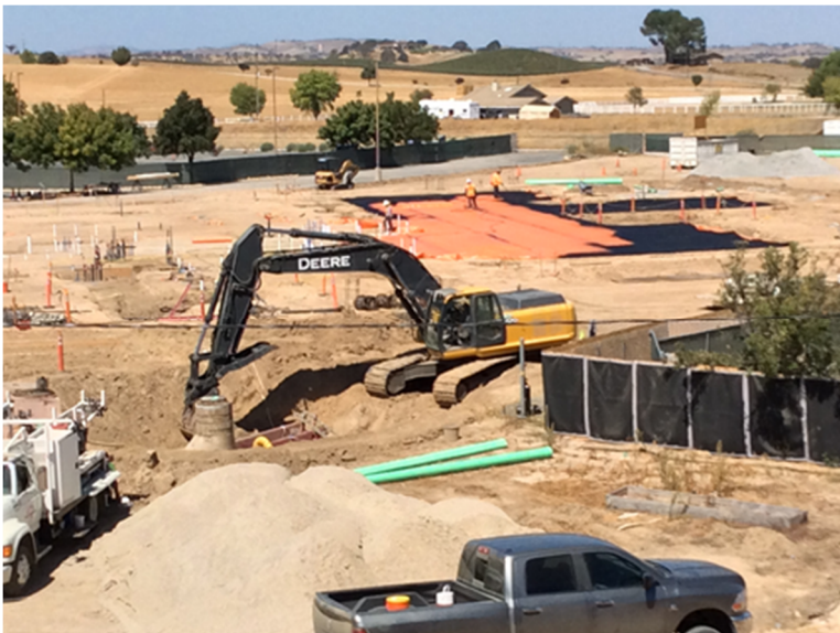
Vapor Barrier Installation & Sanitary Sewer
