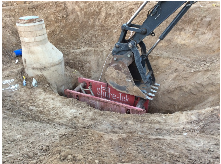
Sanitary Sewer Excavation
