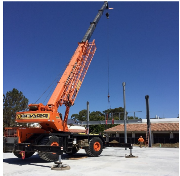
Start of Structural Steel Erection
