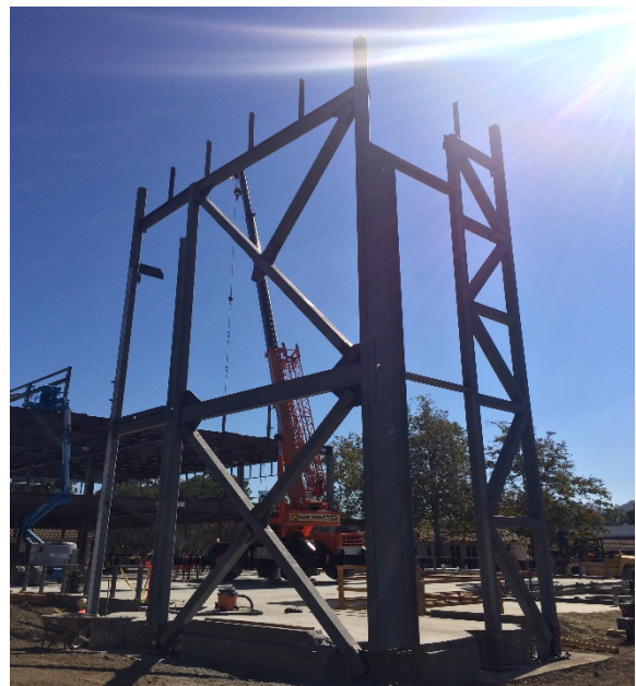
Structural Steel of the Interior Stair Area
