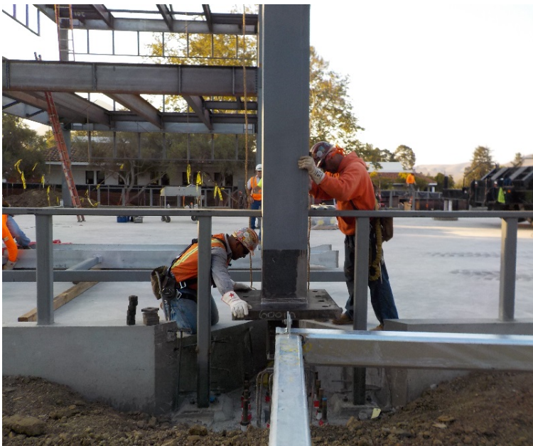
Placing Steel Column
