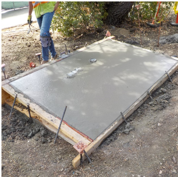
Finished Concrete for New Transformer Equipment
