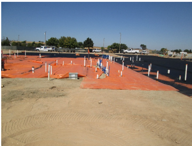
Vapor Barrier Installation
