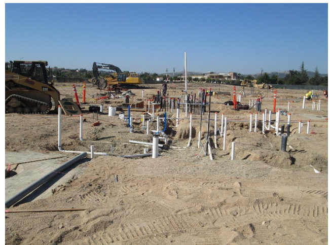
Below Slab Utilities
