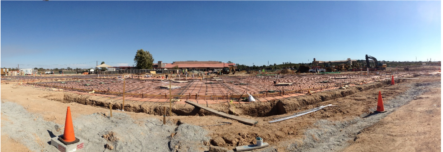
Vapor Barrier and Reinforcement for Concrete Slab on Grade
