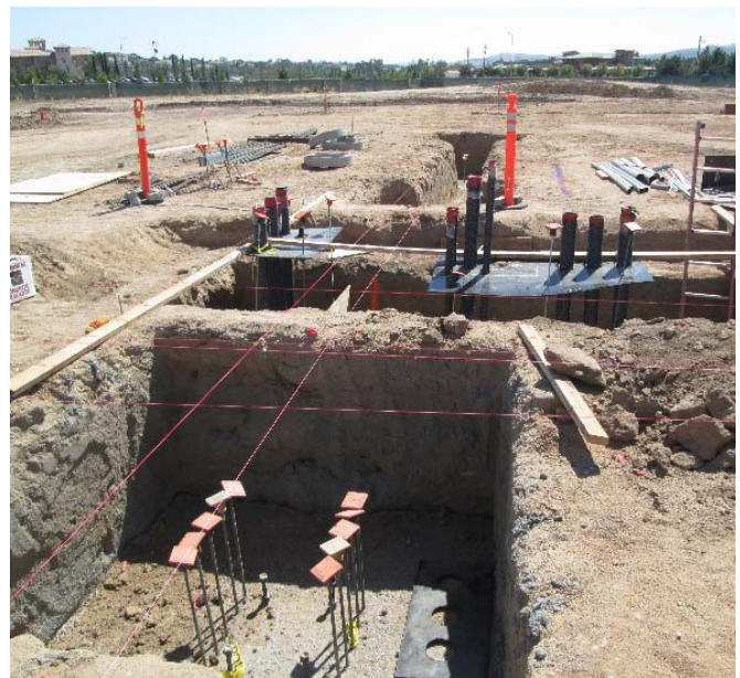
Pad Footing by Deep Electrical
