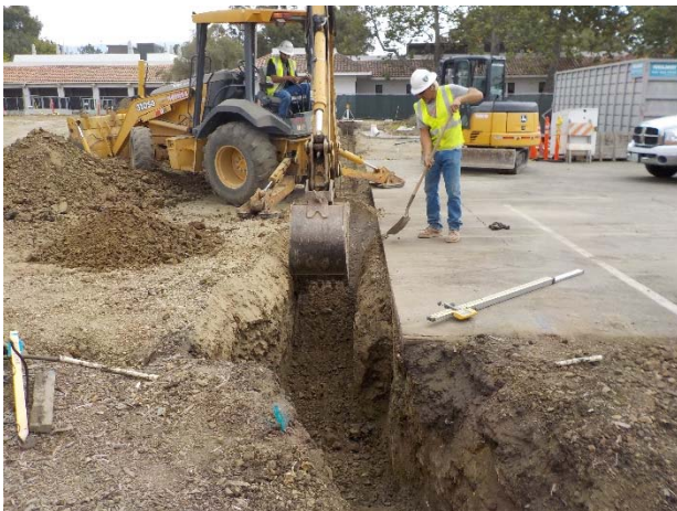
Installation of Storm Drain Piping
