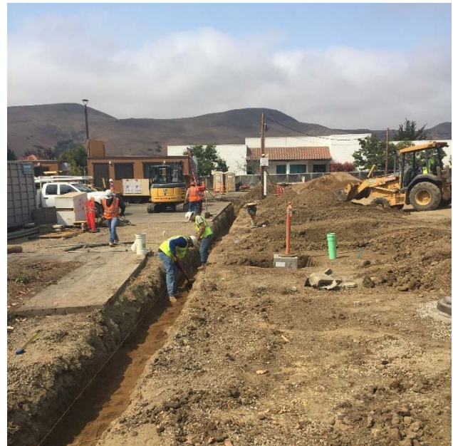
Recompaction of Storm Drain Utilities
