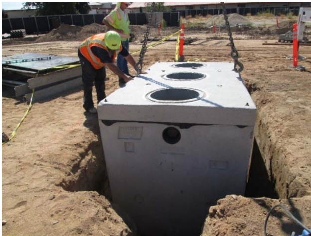
Setting the Grease Interceptor
