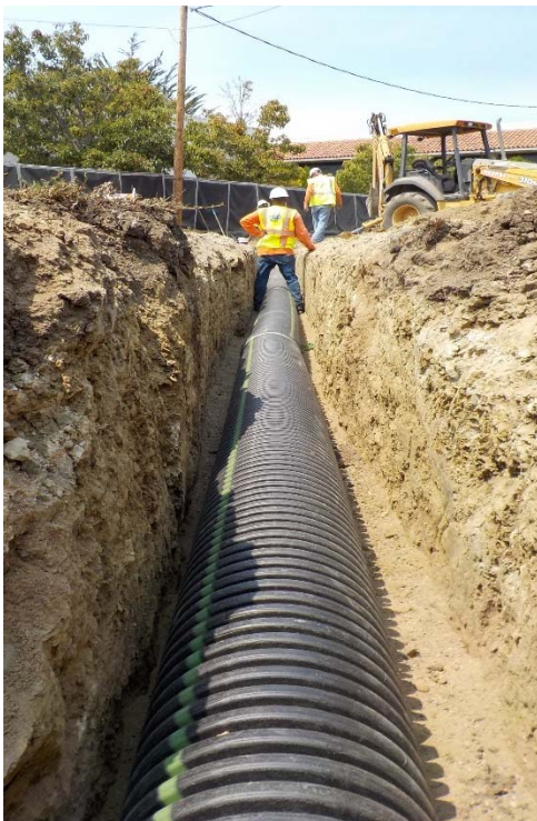
Installation of Storm Drain Utilities
