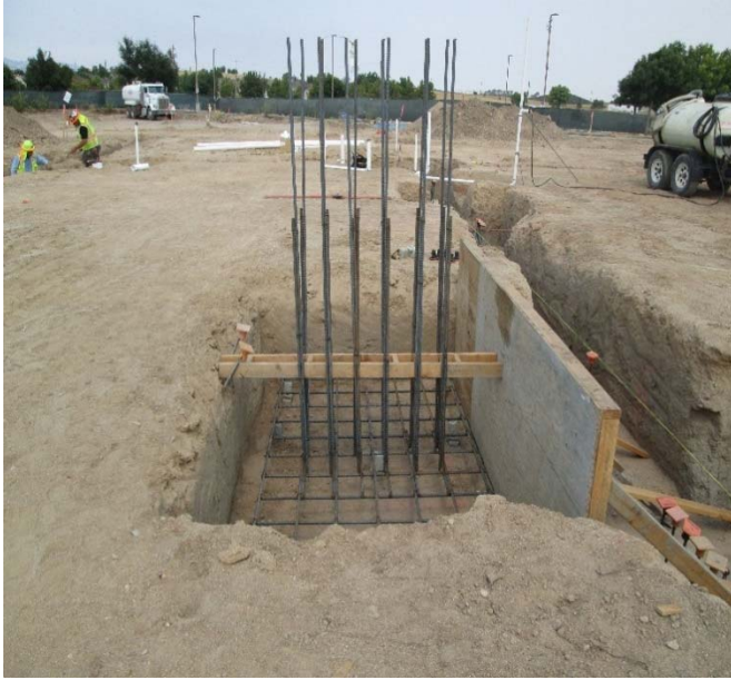
Stair Footing Rebar Installation
