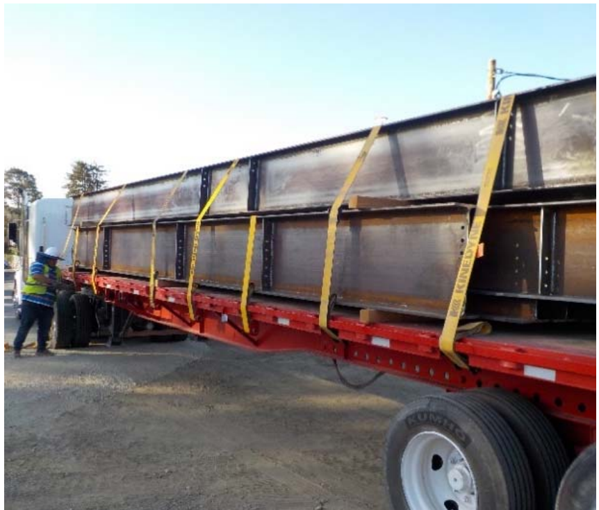
First Delivery of Structural Steel
