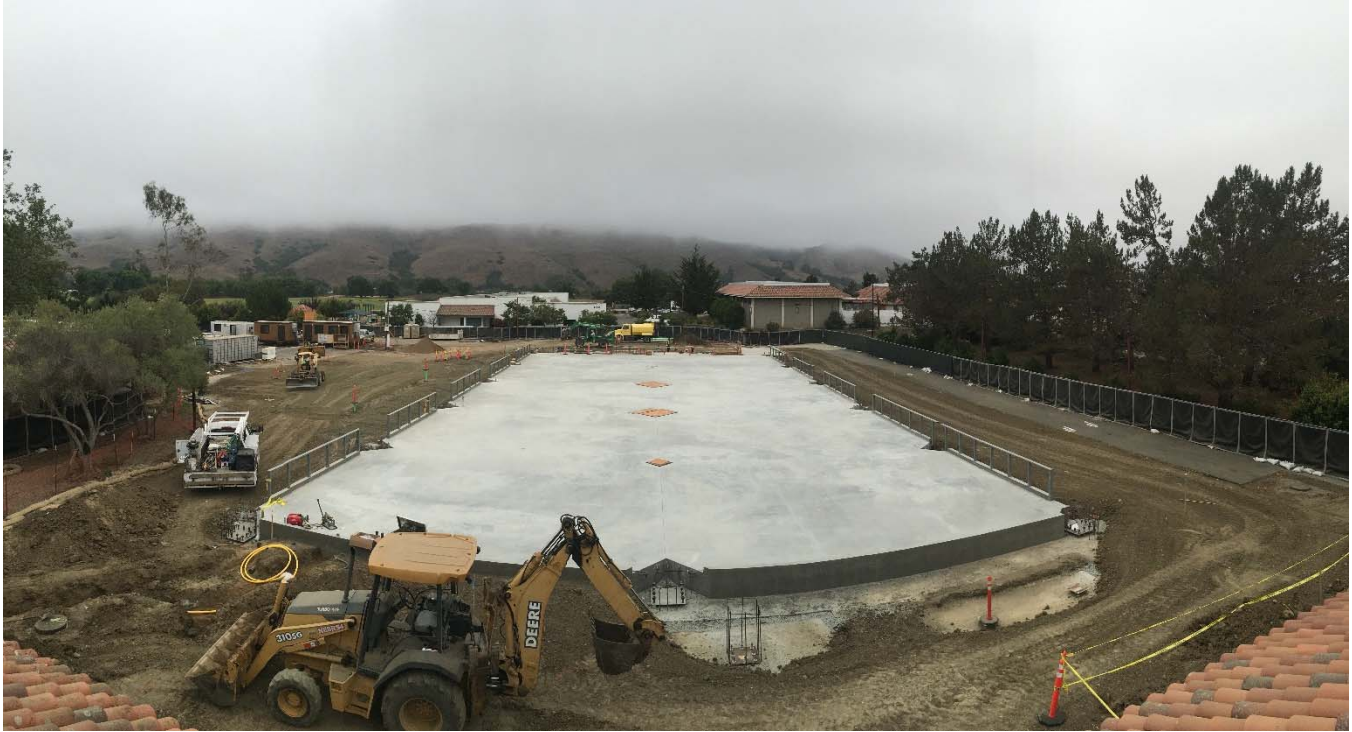
View of the Project from Adjacent Rooftop
