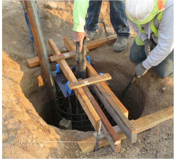
Trellis Footing Anchor Bolt Placement
