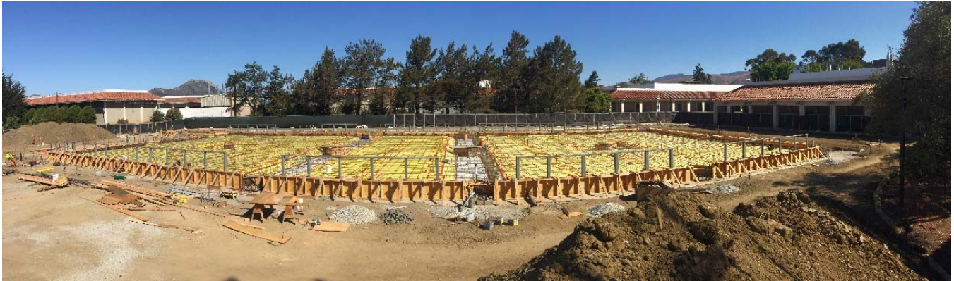
Vapor Barrier Installation Complete with Screed Pins Set and Ready for Concrete Placement
