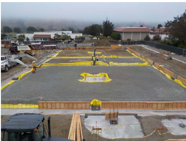
Non-expansive Fill below Slab-on-Grade
