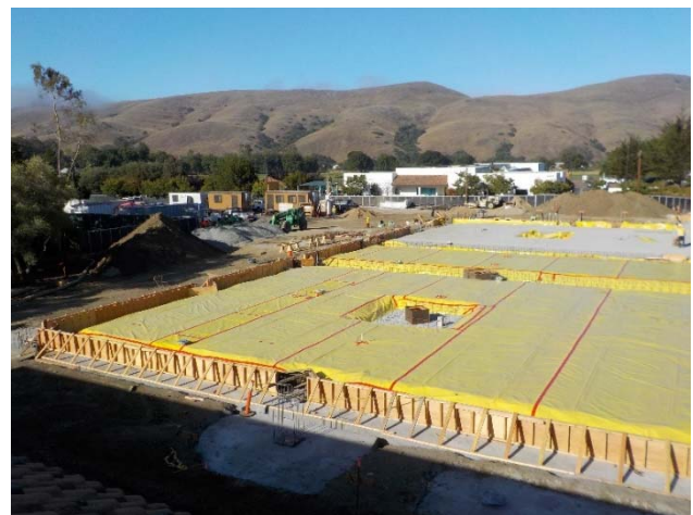
Below-Slab Vapor Barrier Installation at 60%
