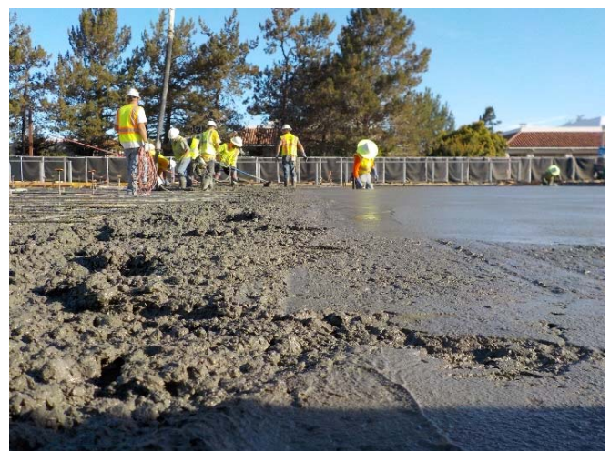
Placement of Concrete for Slab-on-Grade
