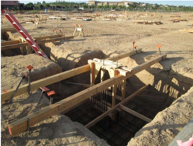
Rebar and Anchor Bolt Installation
