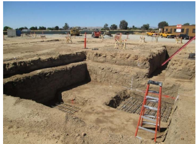
Excavation of the Elevator Pit and Adjacent Pad Footings
