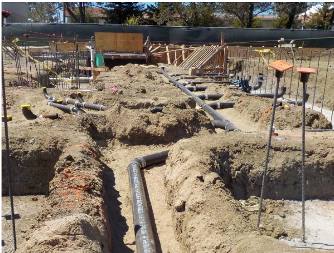
Early Stages of Underground Plumbing Utilities for the Bathrooms
