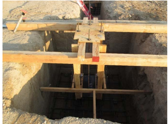
Rebar and Anchor Bolt Installation
