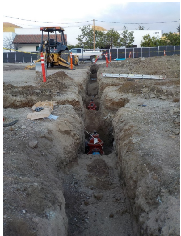
New Site Domestic and Fire Water Line
