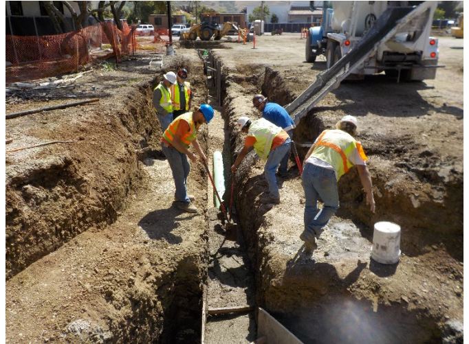
Slurry Backfill over New Sewer Line
