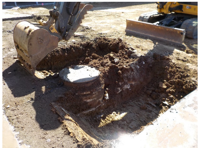
Slurry Backfill over New Sewer Line
