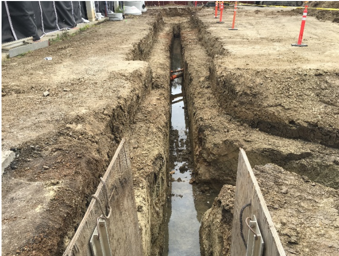
Trench for New Sewer Line
