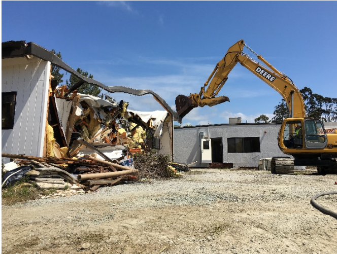
Building Demolition Continued
