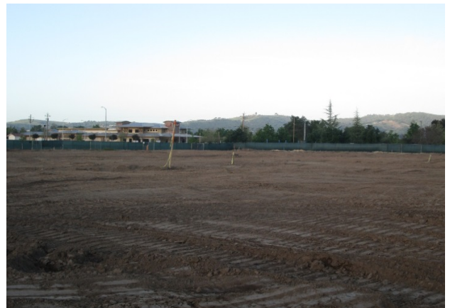
Backfill Operation Completed
