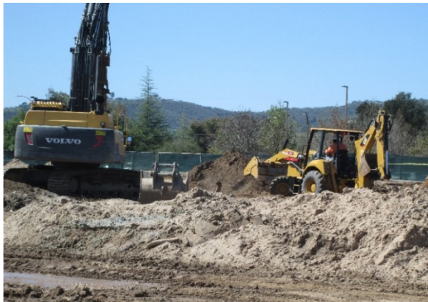
Excavator and Backhoe for Utility Backfilling Operation
