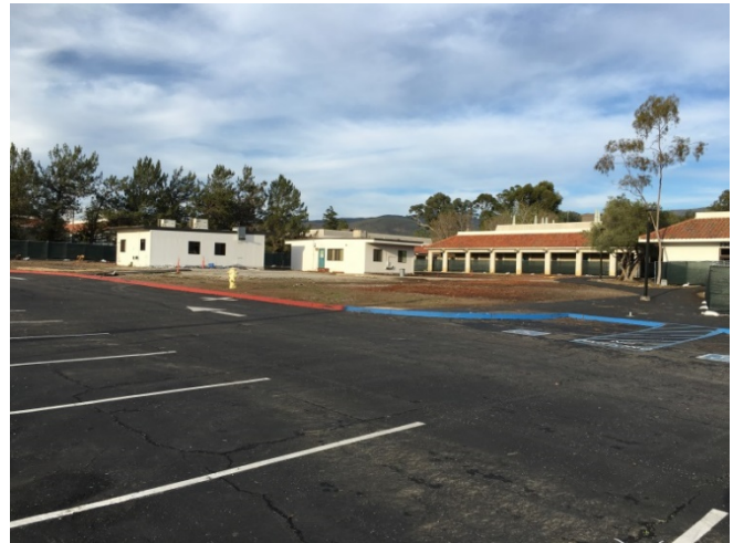
Remaining Portable Buildings
