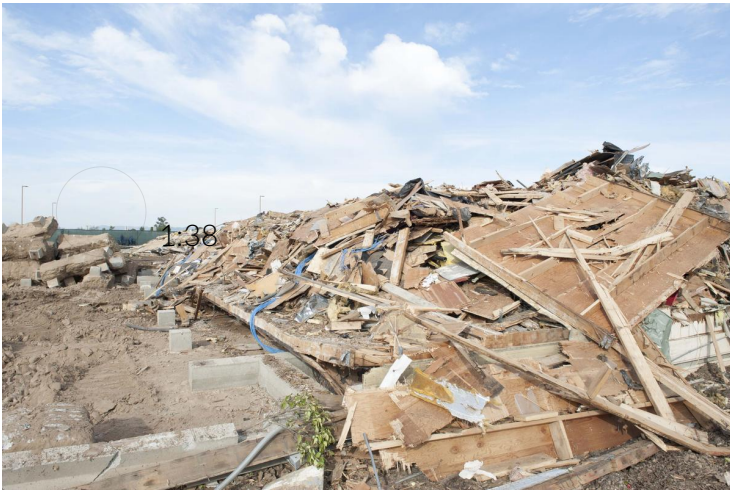
A pile of rubble on the North County Campus following demolition of the temporary classrooms.
