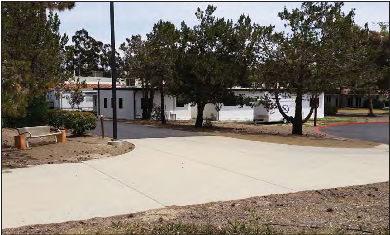
Photo 2: Taken from immediately northwest of the northwestern site boundary, adjacent to the existing parking area, facing southeast.
